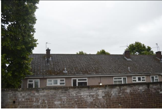
Photograph 7: B7 northern elevation.
