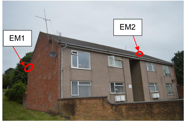
Photograph 4: Example of building B1 – B6 southern and western elevations (using B1 as an example) with emergence feature details.
