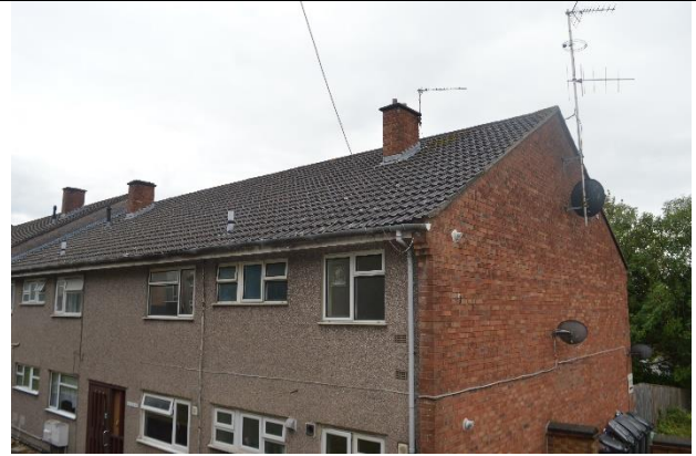
Photograph 8: B8 northern and western elevation.
