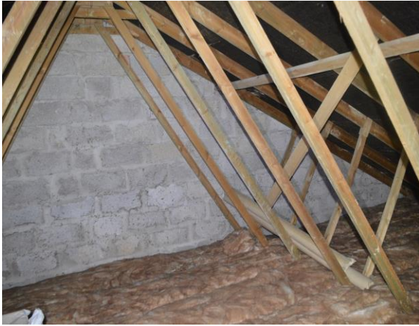
Photograph 1: Example of void interior buildings B1 – B11.
