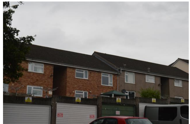
Photograph 10: B9 southern elevation.
