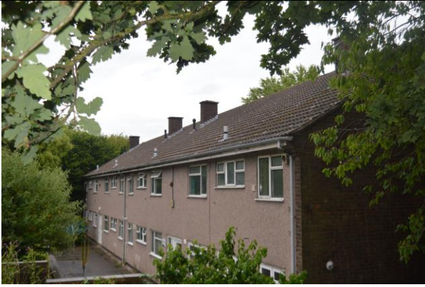
Photograph 15: B11 northern elevation.
