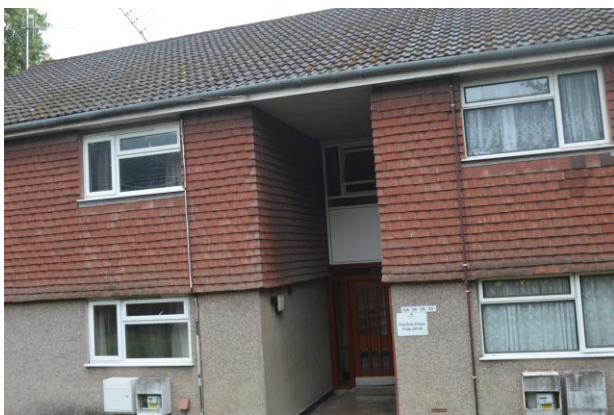
Photograph 11: B9 northern elevation.
