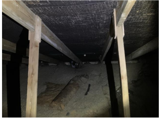
Photograph 2: Example of void insulation, unbind cellulose insulation buildings B1 – B11.
