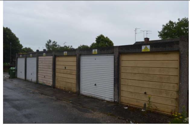
Photograph 16: Exterior of garages.
