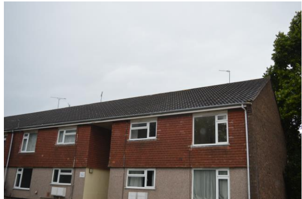
Photograph 6: B7 southern and eastern elevations.
