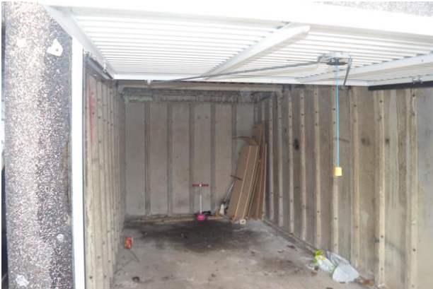
Photograph 17: Interior of garages.
