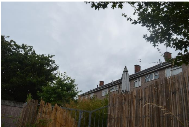
Photograph 9: B8 southern elevation.
