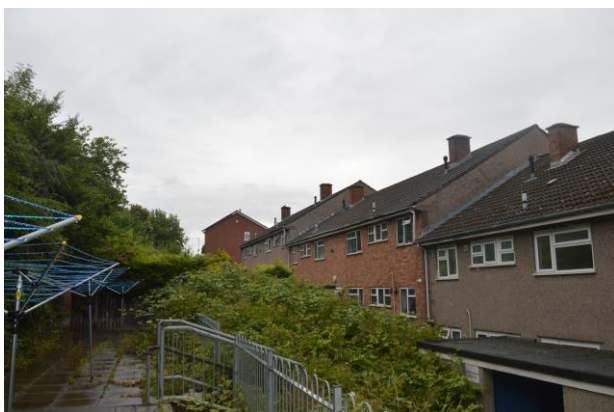
Photograph 13: B10 northern elevation.
