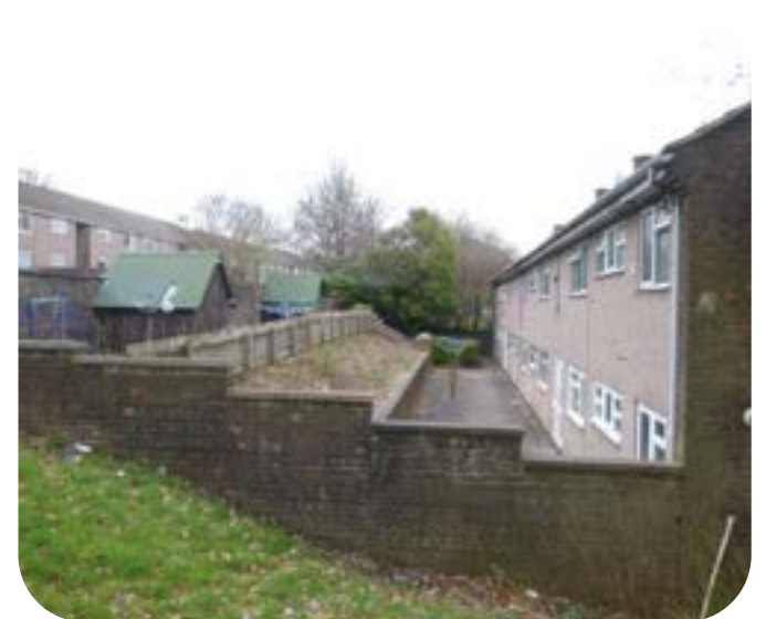
Showing steeply sloping gardens and retaining walls to the rears of the flats
