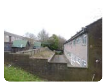
Showing steeply sloping gardens and retaining walls to the rears of the flats.
