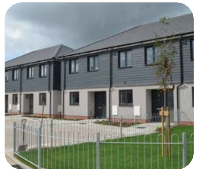
Example of completed Bromford regeneration scheme
