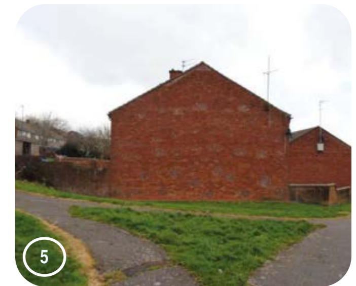
Side wall of the houses next to the park which have no windows overlooking the adjacent footpath. Ideally new homes would have windows to avoid blank side walls and overlook pedestrian routes.
