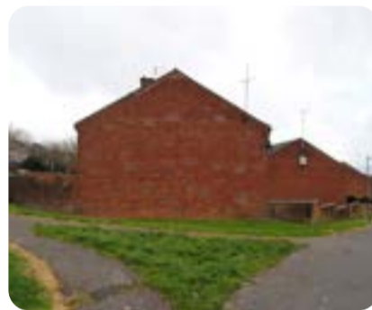
Side wall of the houses next to the park which have no windows overlooking the adjacent footpath.
