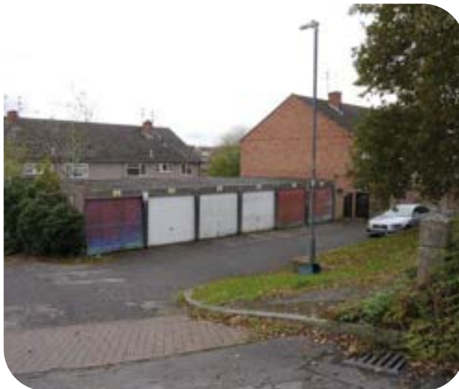
Existing garages proposed for demolition as part of the regeneration of the area
