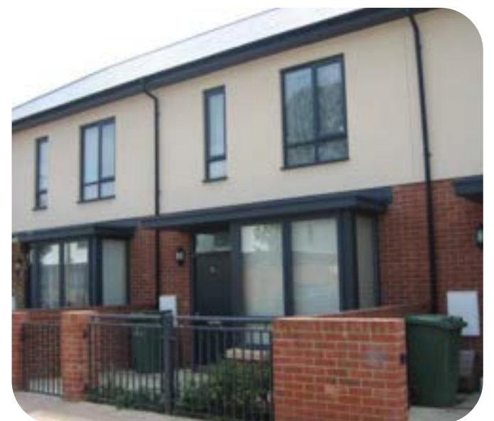
Three and four bedroom houses designed by Nash Partnership. Front garden walls are designed to hide the bins and provide private secure space at the front of the new homes.
