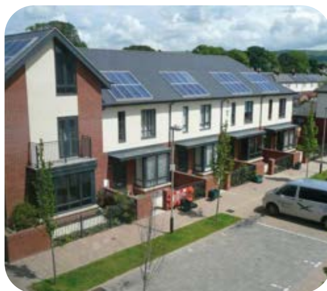
Three and four bedroom houses designed by Nash Partnership. Bay windows provide large areas of south facing glazing and ensure that the pavements and parking areas are well overlooked.
