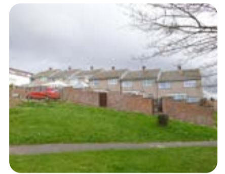
Rear garden wall of the houses that remain backing onto the site. This photo demonstrates how steep the site is in places.
