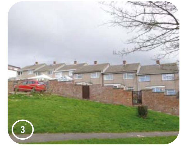
Rear garden wall of the houses that remain backing onto the site. Rear garden access to these homes will be retained in the proposed layout. This photo demonstrates how steep the site is in places.
