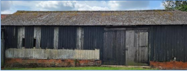
Barn 4 from the north and internal view to show the construction
