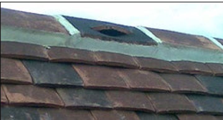
c) Made by Tudor Roof Tiles ( www.tudorrooftiles.co.uk ) this 'top tunnel' tile provides a tunnel to an entrance hole in the undertiles, allowing bats to crawl into a roost or along the ridge beam where a cavity has been created.
