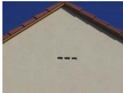
e) Schwegler 1FR Bat Tube, to be integrated into building wall, and either bricked in or rendered. Self cleaning. Dimensions: 47.5 x 20 x 12cm.
