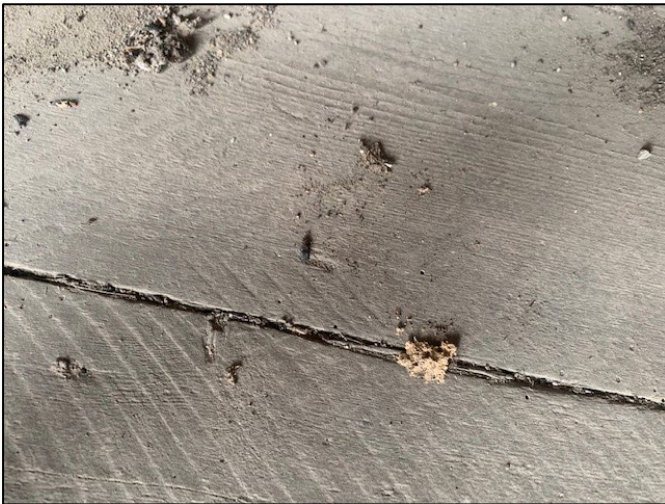
e) B1, bat dropping found on stairs leading up to mezzanine.
