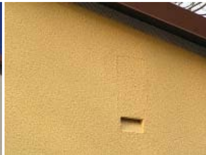
e) Schwegler 1FR Bat Tube, to be integrated into building wall, and either bricked in or rendered. Self cleaning. Dimensions: 47.5 x 20 x 12cm.
