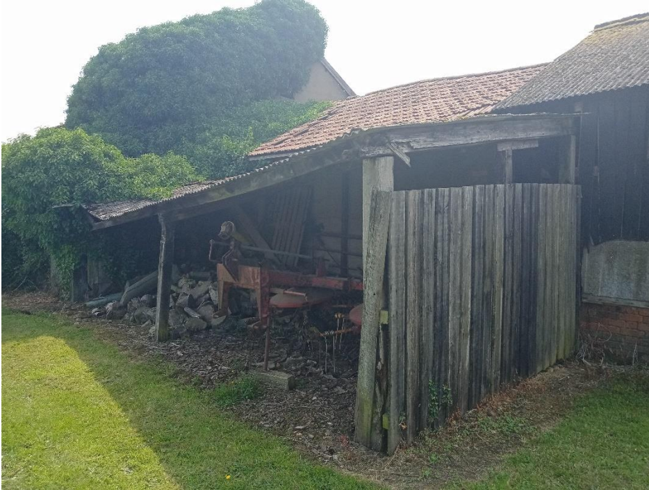
Fig 15. View of timber structure to the front of Barn 3
