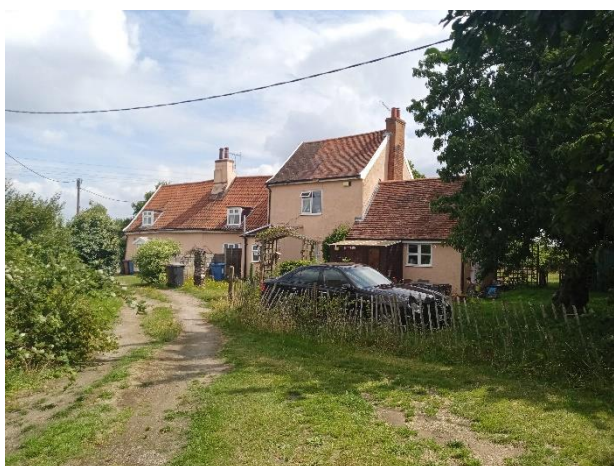
Fig 21. Rear elevation of Potash Farm Cottages
