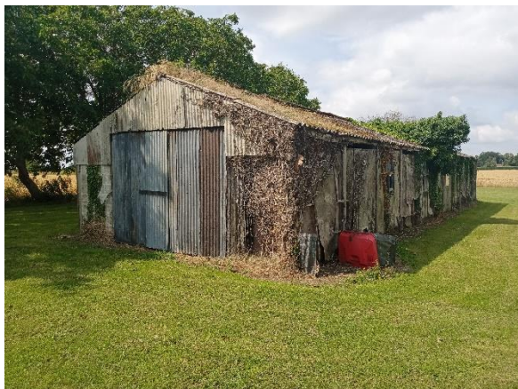
Fig 19. Former WW2 building to the South of the site
