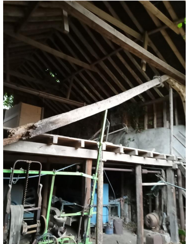
Fig 8. Threshing Barn 1. West bays with existing mezzanine level
