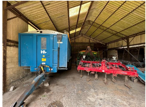
Fig 13. Modern steel framed barn 2, Internal view.
