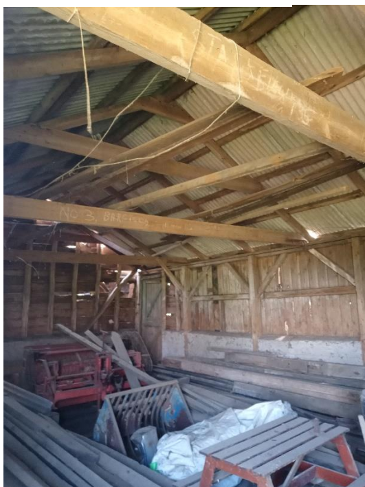
Fig 18. Internal view of Barn 4. Note modern studwork.
