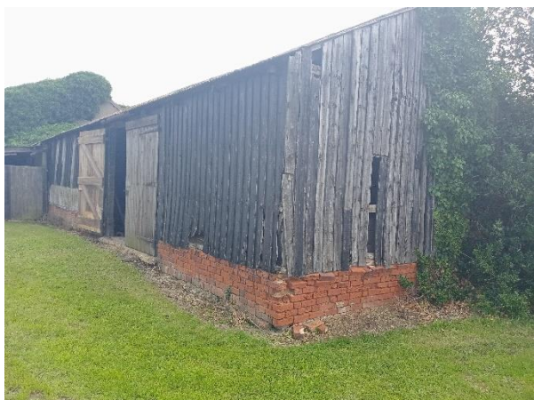
Fig 16. North-West view of Barn 4.
