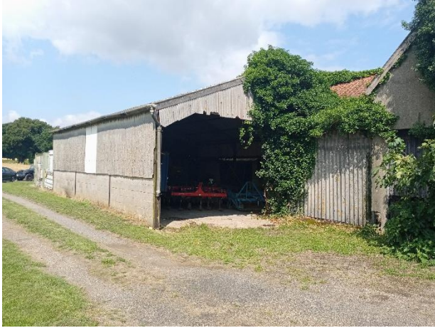
Fig 10. Modern steel framed barn 2, east elevation.
