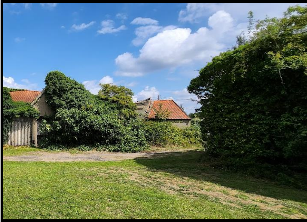
Building 9 is under the foliage in the right of the picture.
