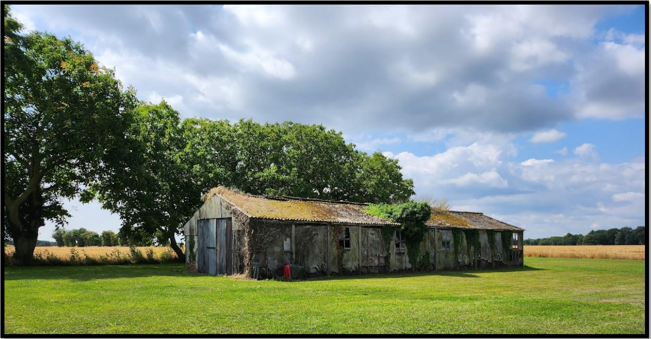
Building 8 viewed looking South Westerly.
