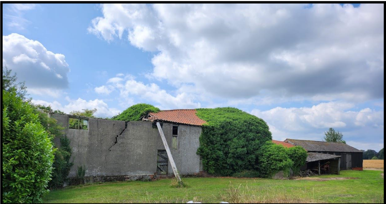
The North elevation exterior facing Southwest.
