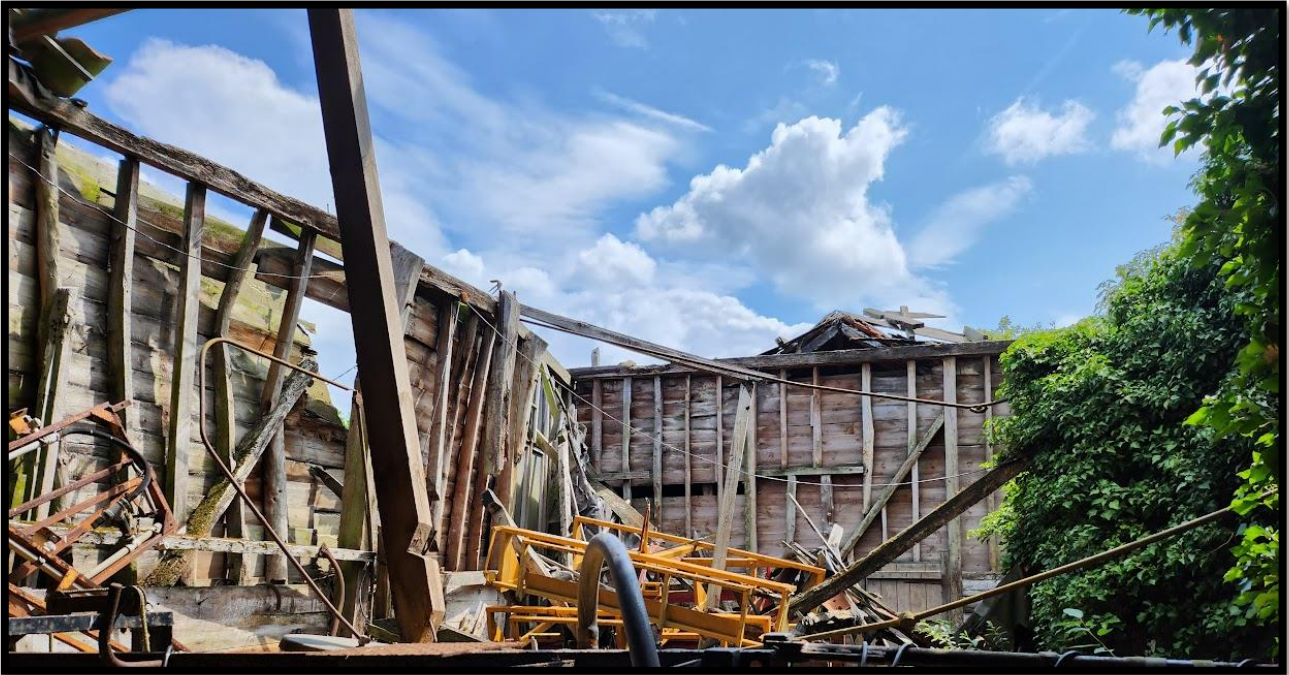
The interior facing East from the centre of the building.
