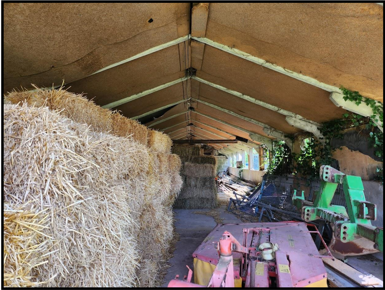
Interior view of building 8.
