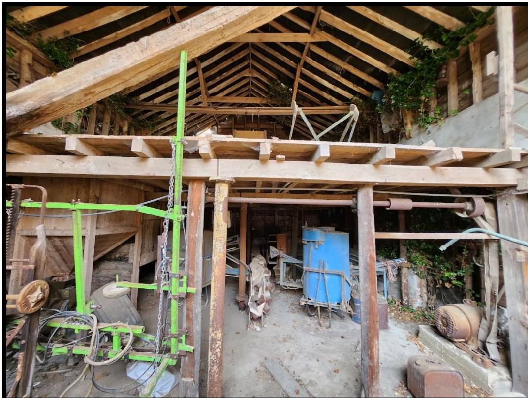
In the image above we see the start of the remaining roof, a C20 replacement that has catastrophically failed. A timber mezzanine floor has also been installed on the left.
