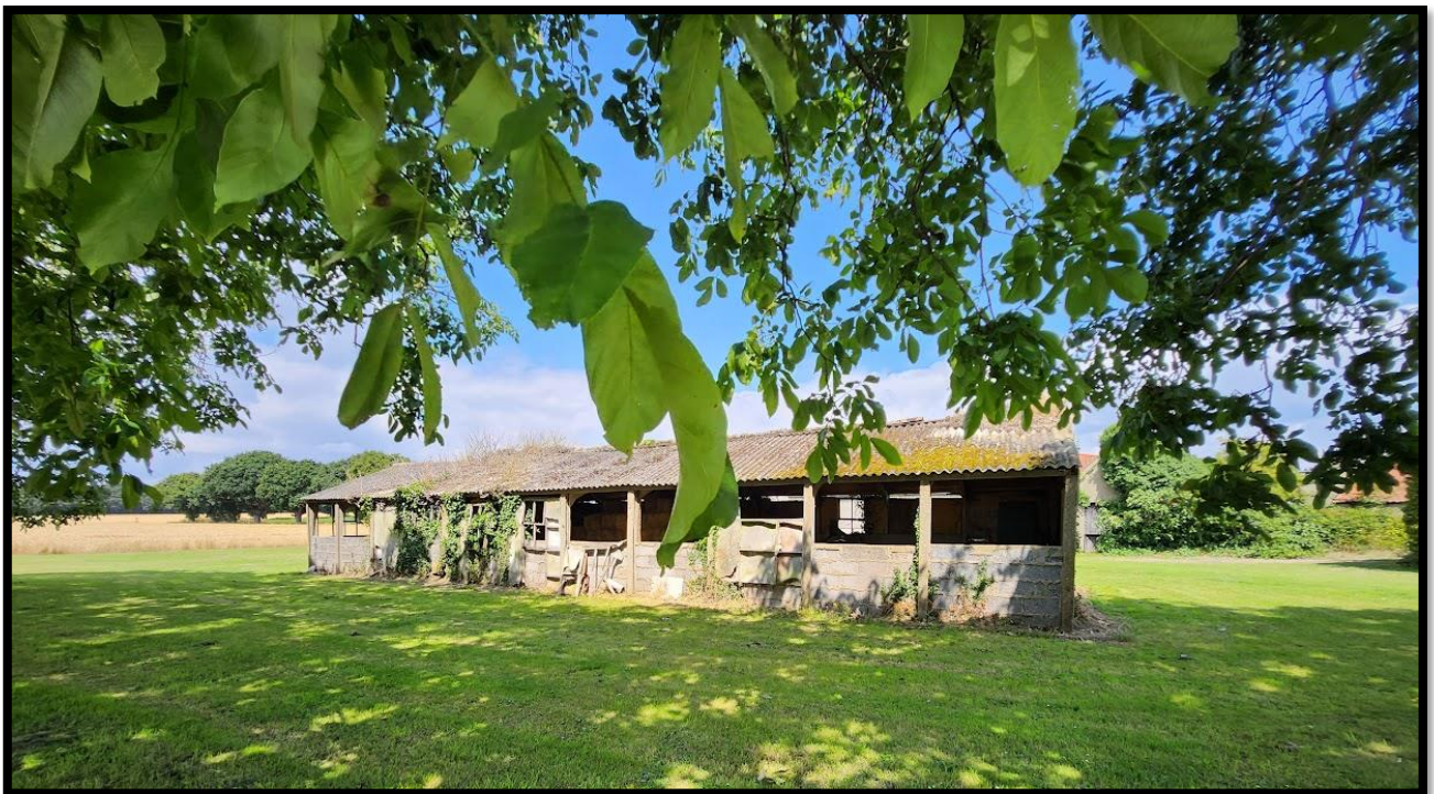
Building 8 viewed looking North Easterly.
