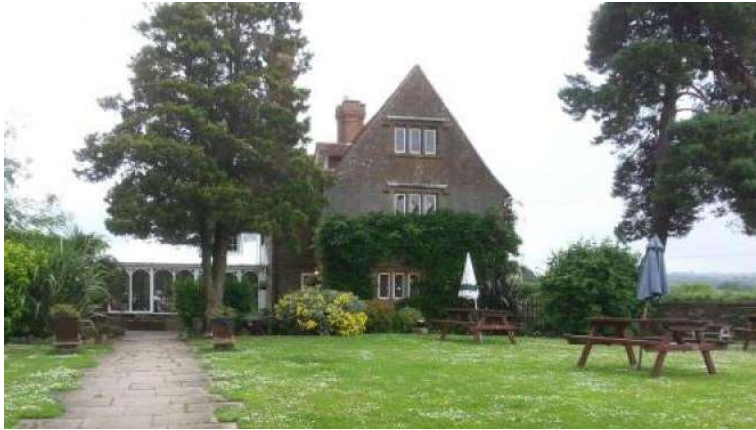
North Elevation showing large modern conservatory
