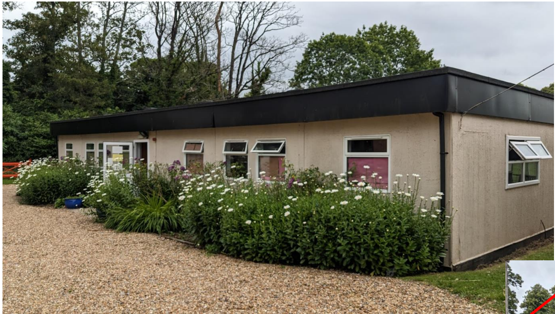
Figure 5. View of western elevation of building 1 and supporting photos of PRFs and eastern elevation (taken July 2023).
