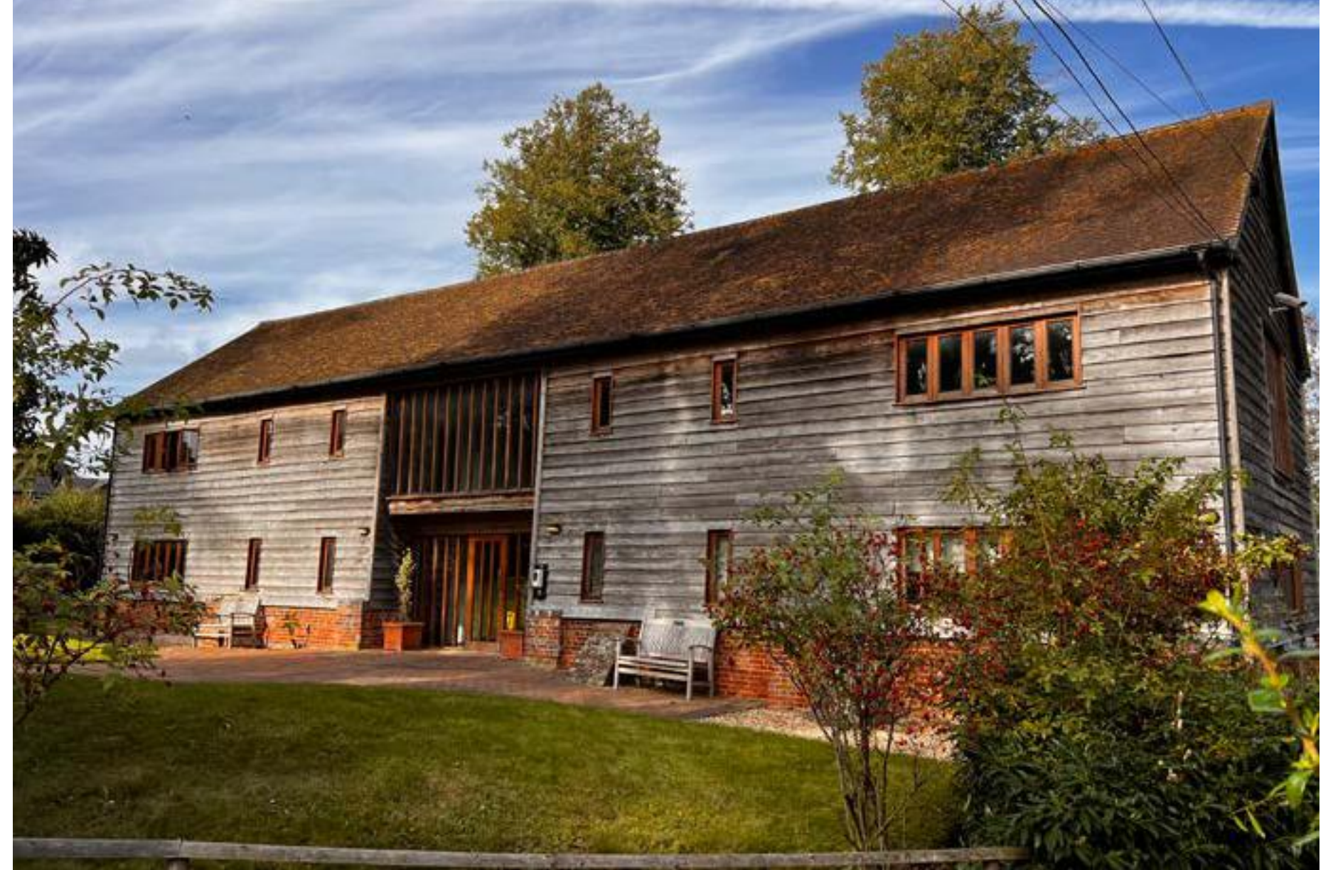
Plate 6: Structure to the west of the modern school buildings that illustrates an agricultural design.
