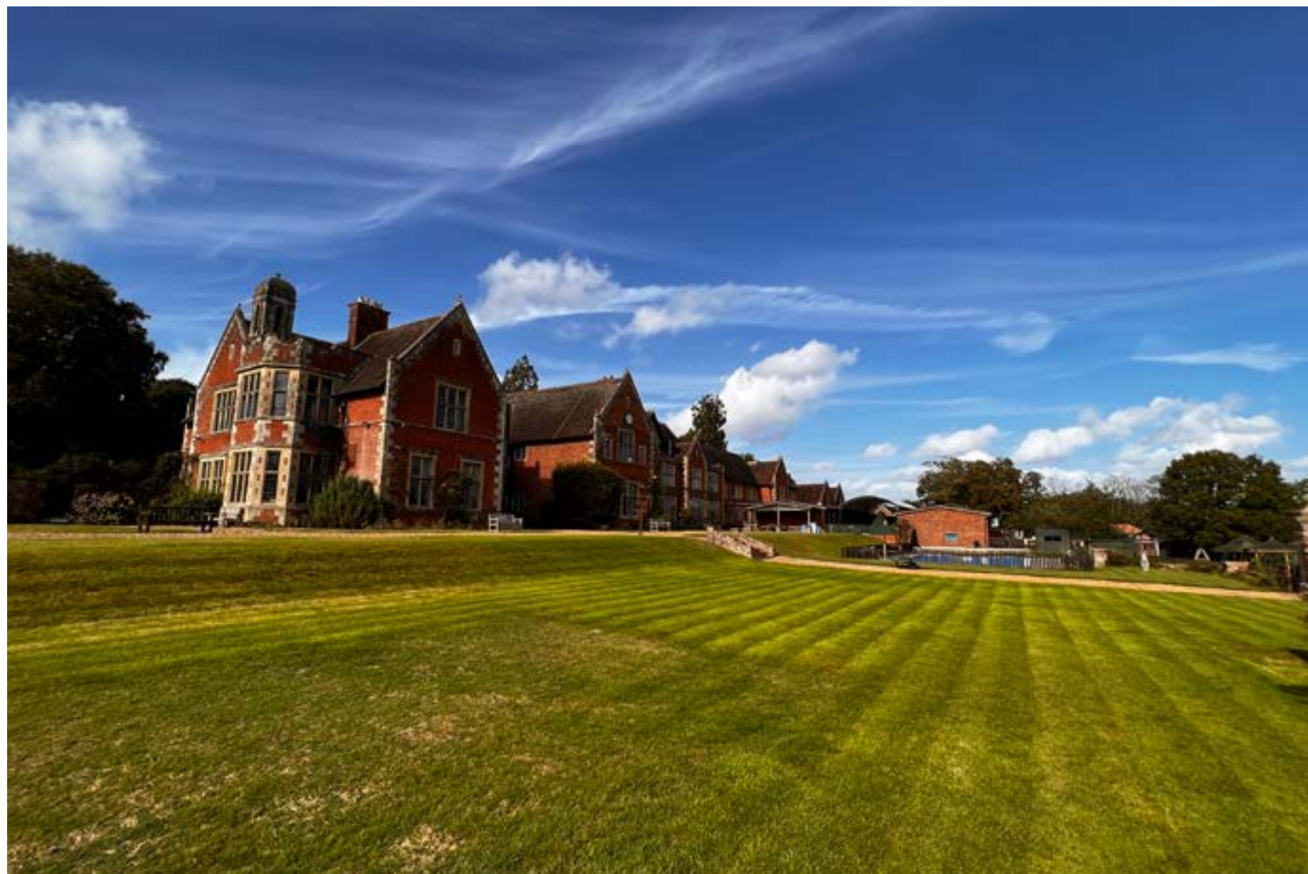
Plate 3: Taken on the terrace to the east of Forres Sandle Manor, looking northwest towards the collection of modern school buildings.
