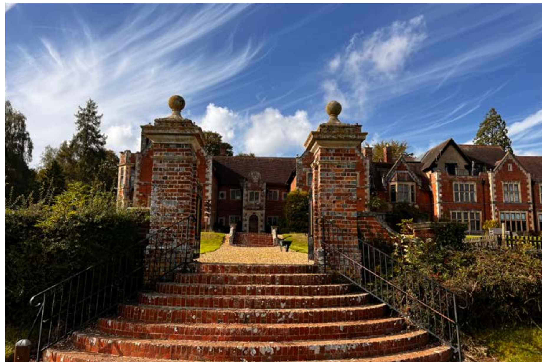
Plate 4: The gate piers leading onto the terrace to the east of Forres Sandle Manor.
