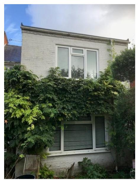
This proposal seeks to add a slate pitched roof to the rear extension, to match the main house, as well as the rear elevation of the adjoining 2 Quay Road which already features a large rear gable, as shown on the elevations. The proposal also seeks to improve the fenestration by changing the existing horizontal rear windows for a canted bay of more traditional form, with improved vertical emphasis.
