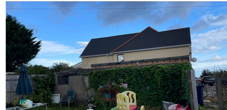
Existing side view of garage & No1A Marshall Road, from 112 Hollow Way garden
