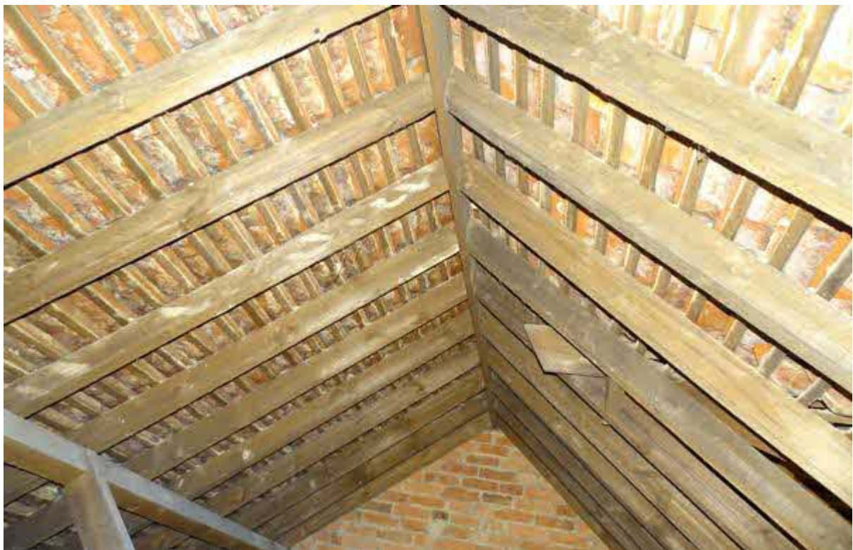
Image 8 – internal view from below the main roof coverings of the property.
