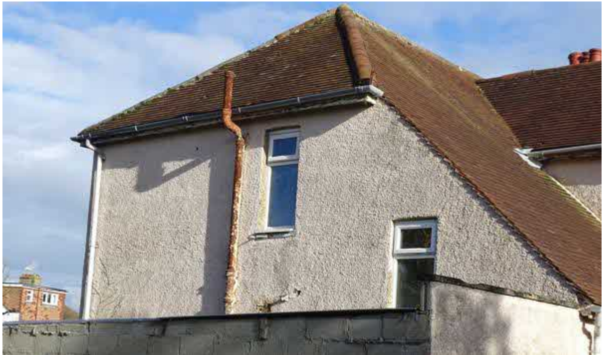
Image 3 – West facing elevation of the structure
