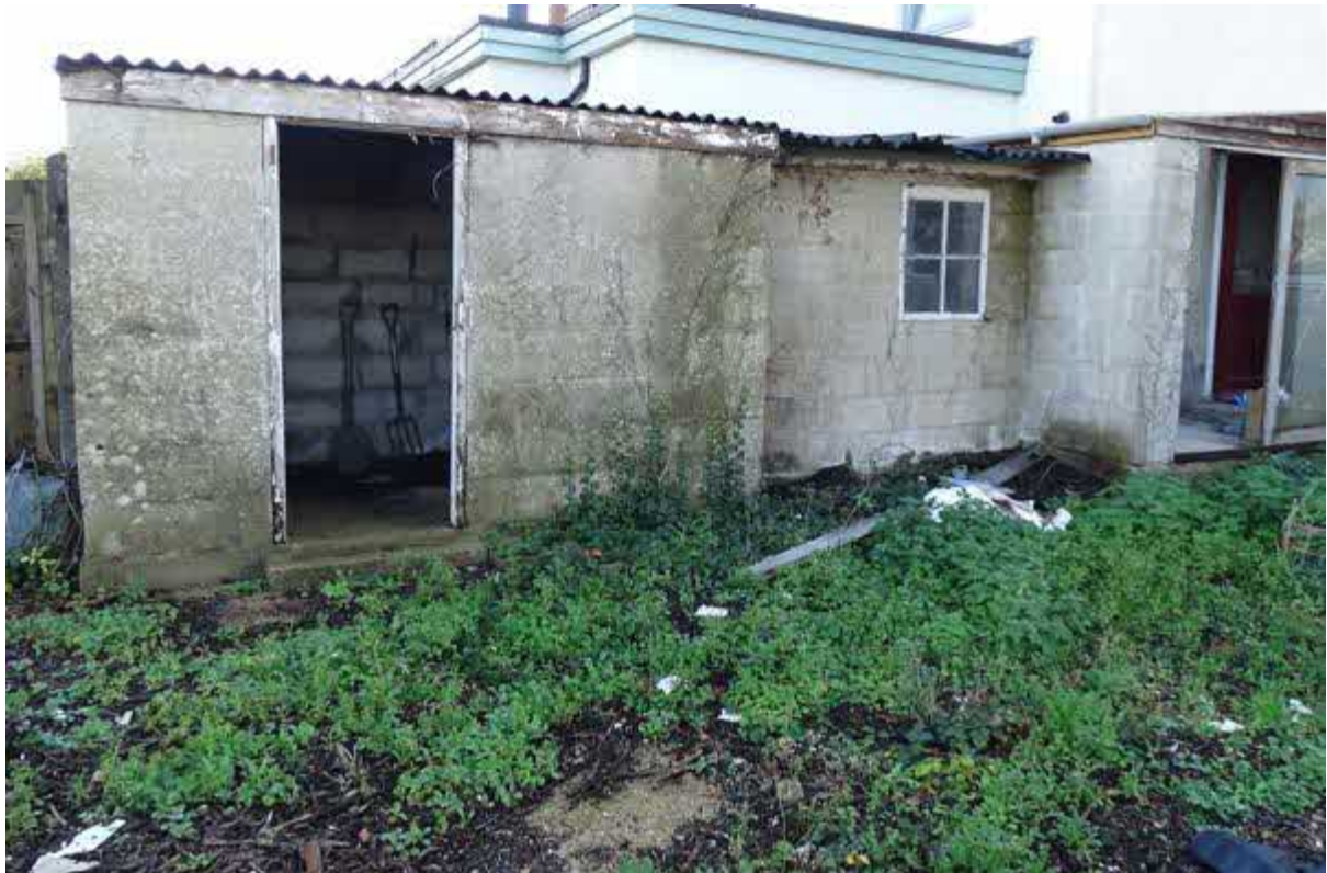
Image 5 – Outbuildings to the rear of the main house which have demonstrated a fabricated flat roof sheet coverings
