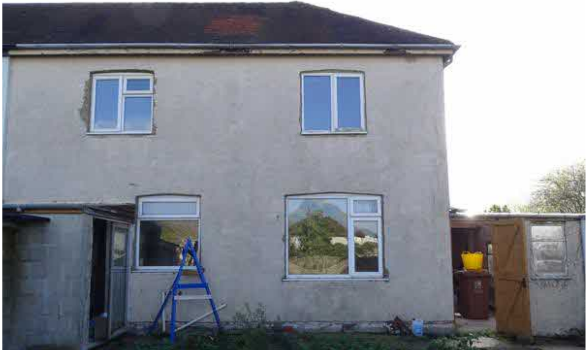
Image 4 – Rear North facing elevation of the structure
