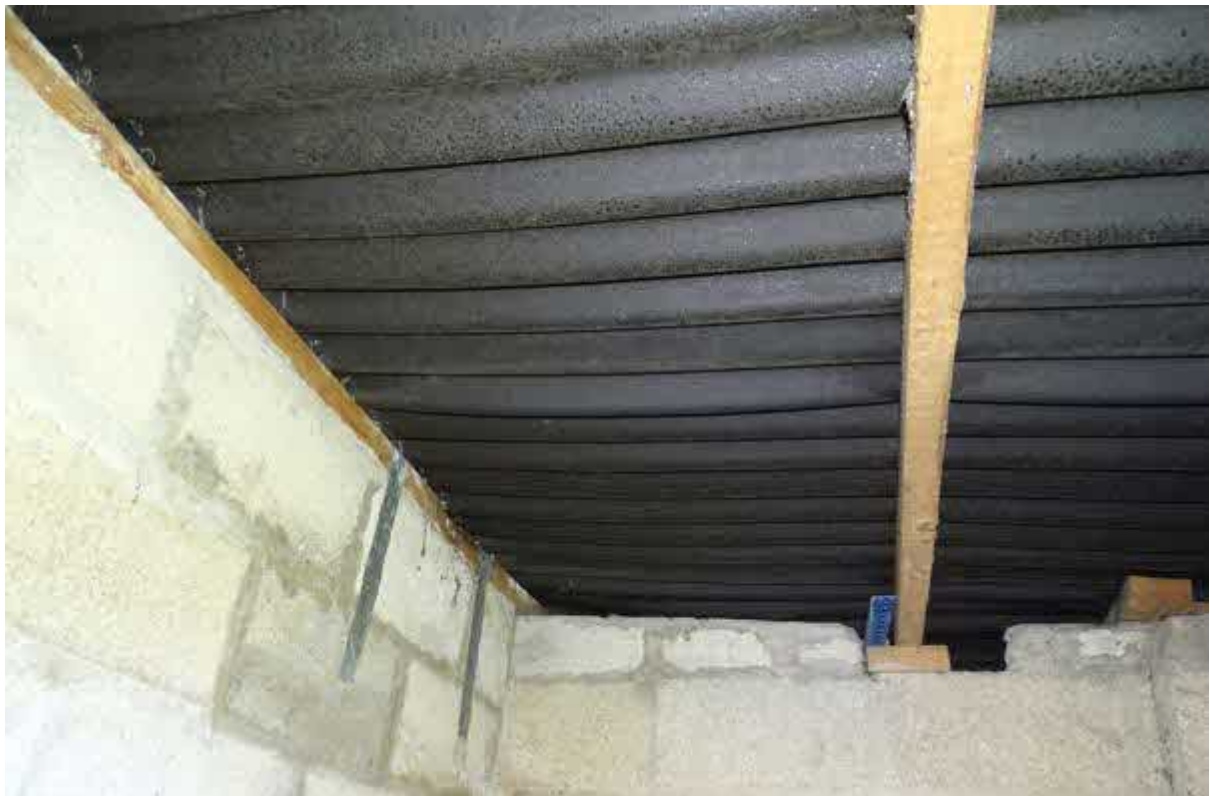
Image 6 – Internal view from within the above outbuildings
