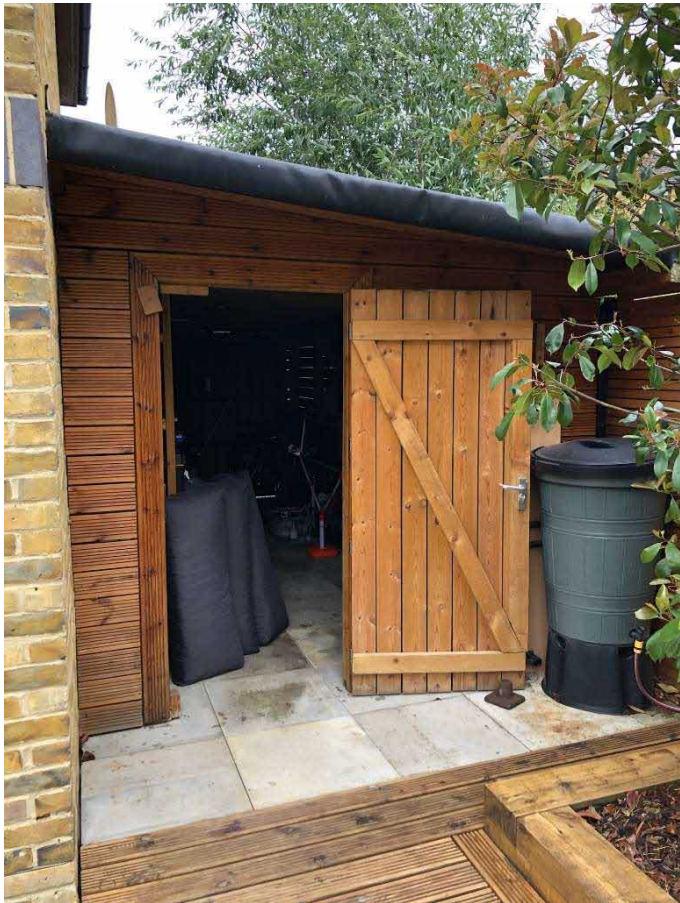
Further context to 15 Blacksmiths Meadow - existing shed –rear view
