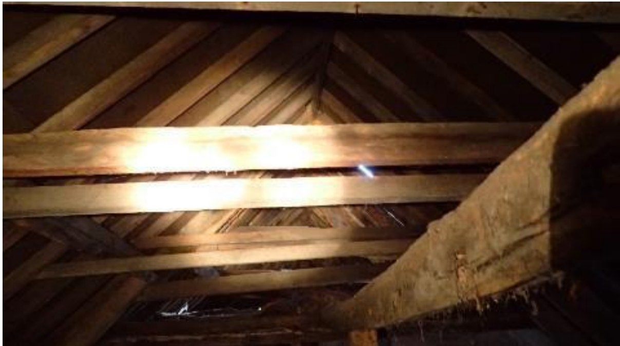
Photograph 7: Interior of attic space of west section of outbuilding
