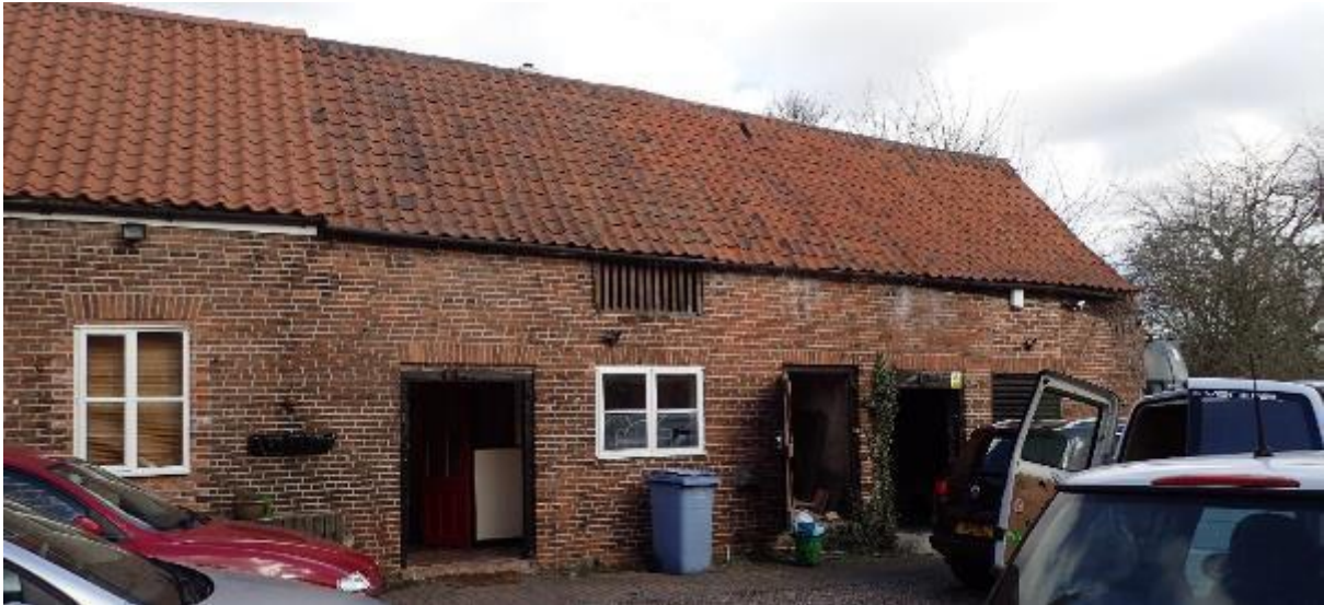
Photograph 5: South aspect of outbuilding attached to east aspect of dwelling
