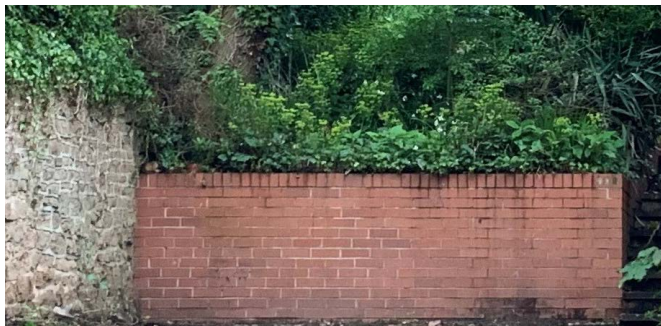
Existing brick wall to rear of garden retained
