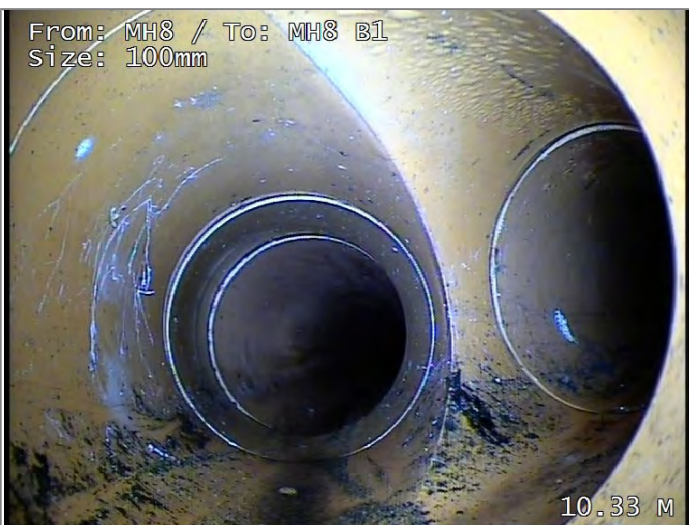
Junction at 3 o'clock, diameter 100mm
