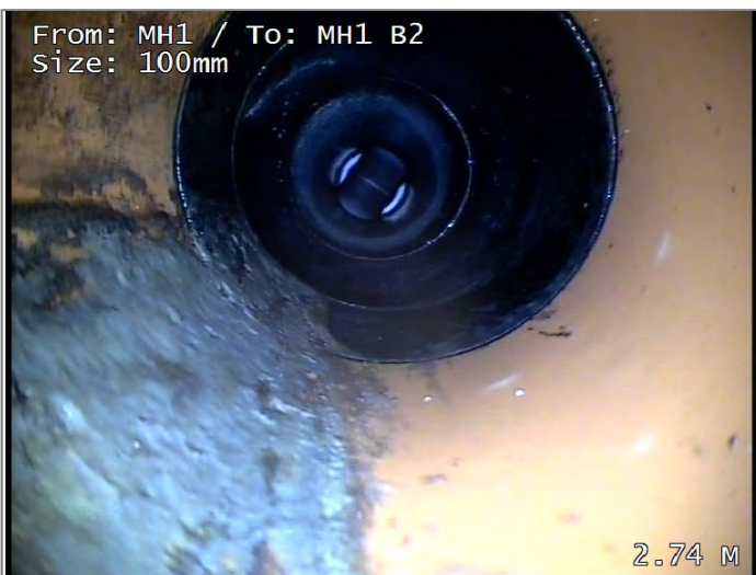
Finish node type, major connection without manhole, reference MH1 B2 REST BEND
