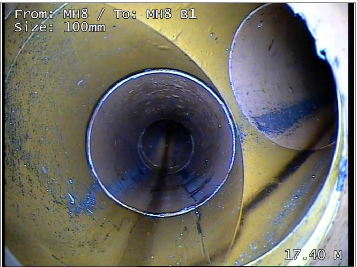
Junction at 2 o'clock, diameter 100mm
