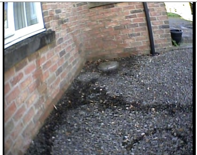
Manhole / Access Point: MH4 Location
