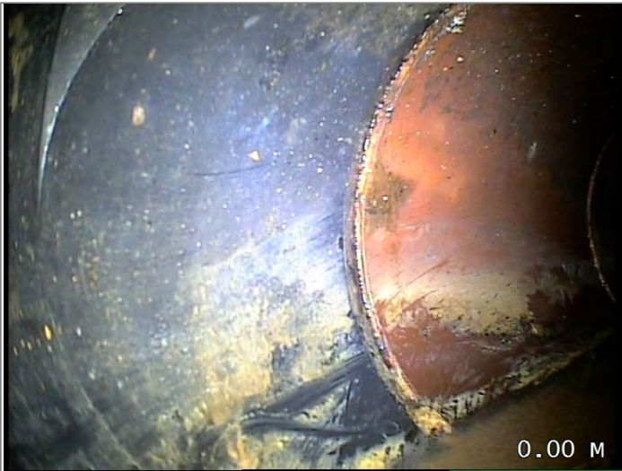
Start node type, inspection chamber, reference MH7 (BURIED)
