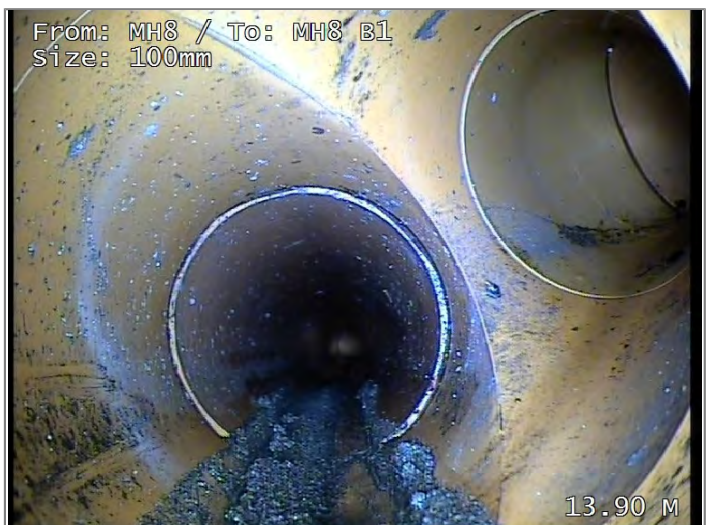
Junction at 2 o'clock, diameter 100mm
