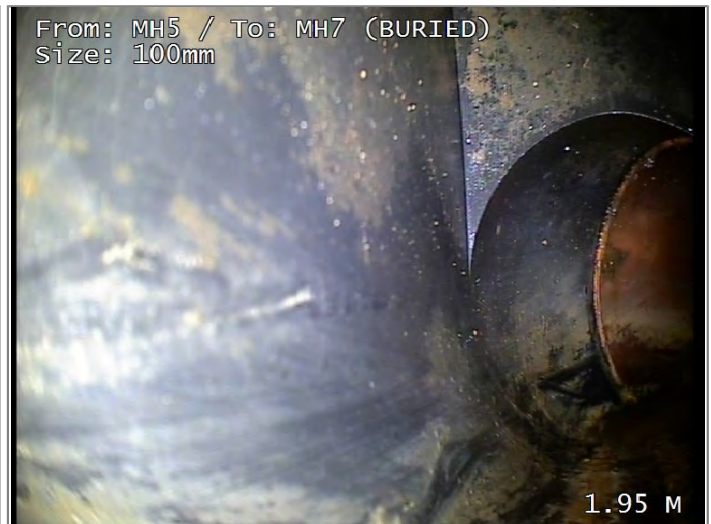
Finish node type, inspection chamber, reference MH7 (BURIED)
