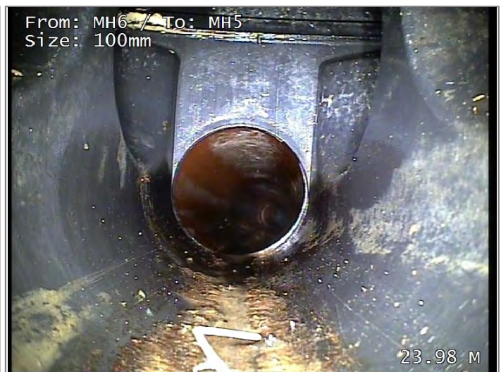
Finish node type, inspection chamber, reference MH5
