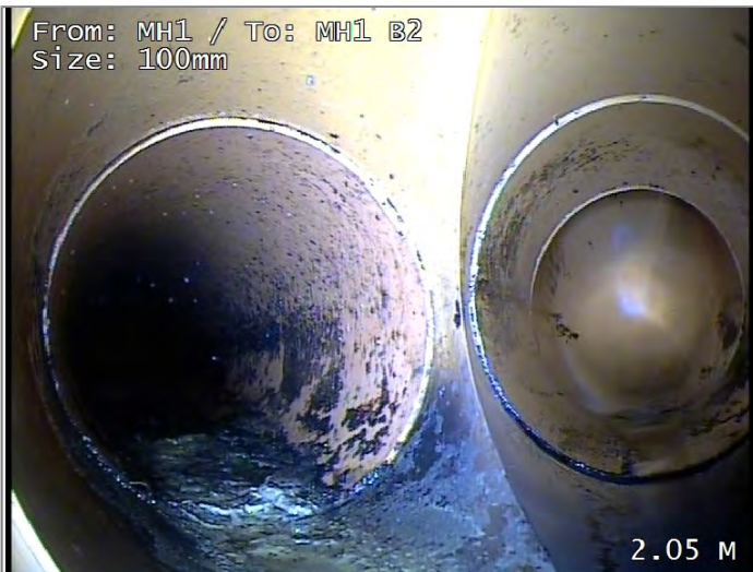
Junction at 9 o'clock, diameter 100mm
