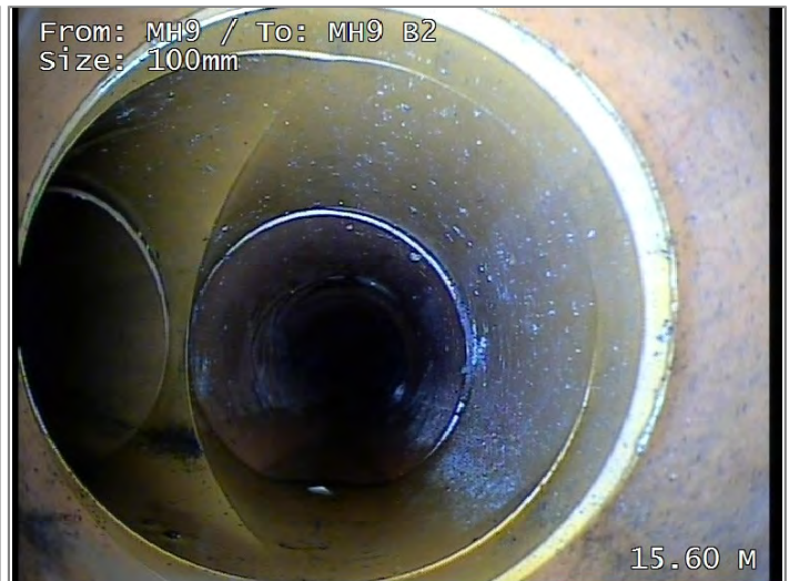
Junction at 9 o'clock, diameter 100mm
