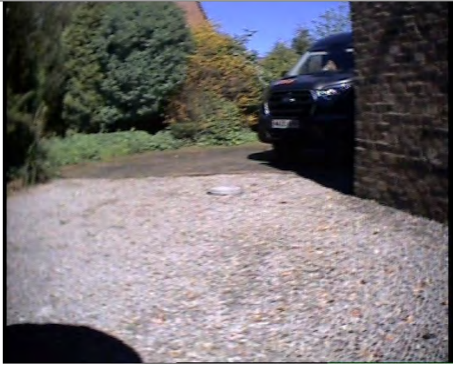
Manhole / Access Point: MH8 Location
