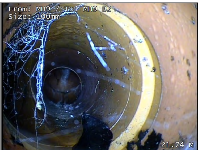
Junction at 9 o'clock, diameter 100mm
