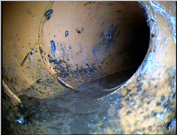
Start node type, manhole, reference MH8
