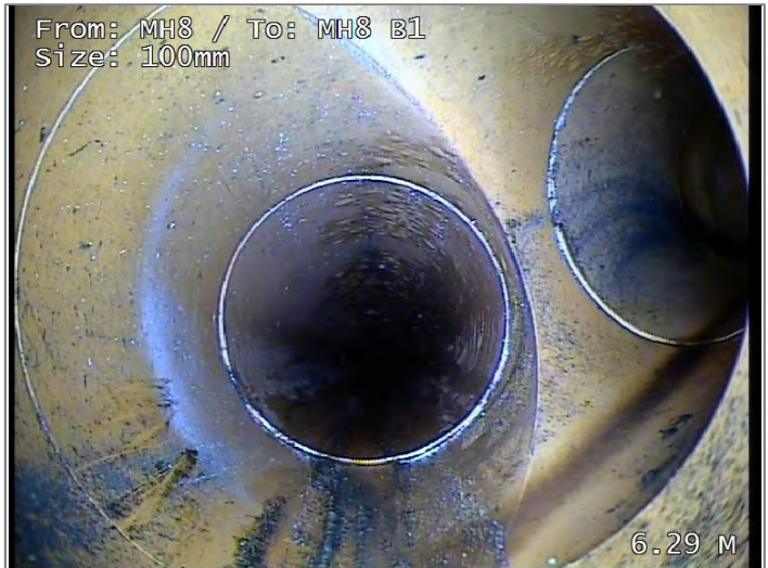
Junction at 2 o'clock, diameter 100mm
