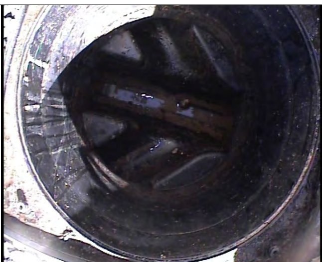
Manhole / Access Point: MH6 Internal
