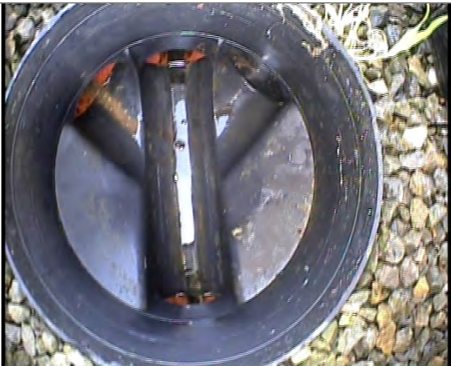
Manhole / Access Point: MH2 Internal
