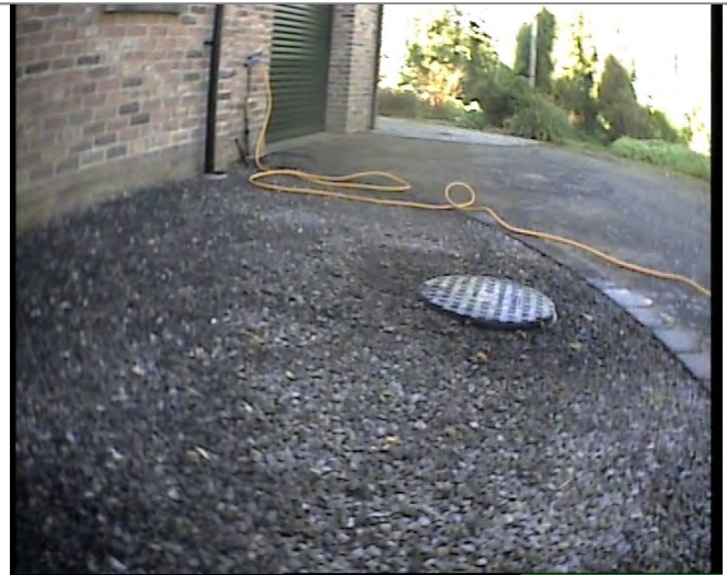
Manhole / Access Point: MH1 Location
