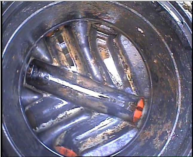
Manhole / Access Point: MH3 Internal
