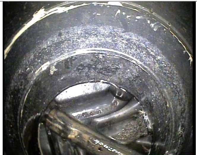
Manhole / Access Point: MH5 Internal
