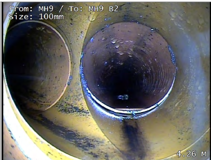
Junction at 9 o'clock, diameter 100mm
