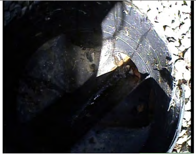
Manhole / Access Point: MH8 Internal
