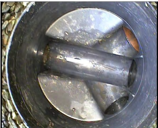
Manhole / Access Point: MH4 Internal
