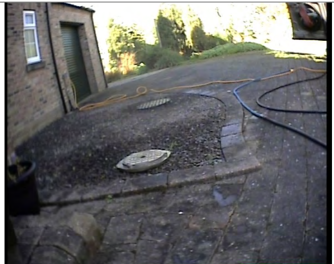
Manhole / Access Point: MH2 Location
