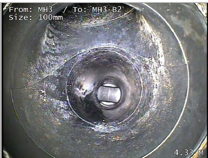
Finish node type, major connection without manhole, reference MH3 B2 REST BEND.
