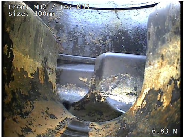
Finish node type, inspection chamber, reference MH3
