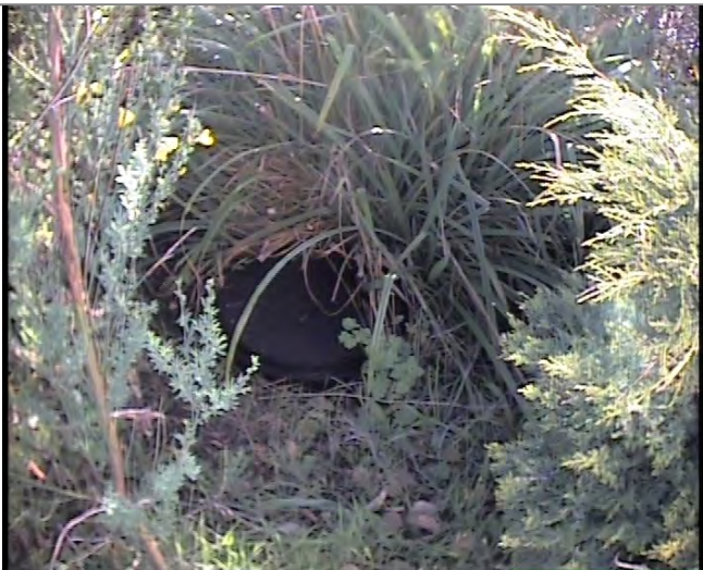
Manhole / Access Point: MH5 Location
