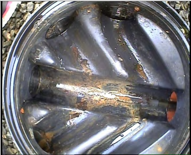
Manhole / Access Point: MH1 Internal
