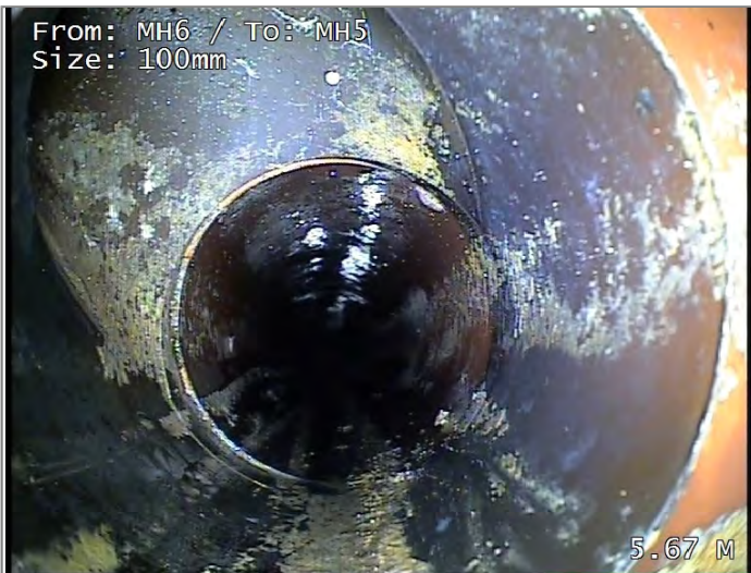
Junction at 11 o'clock, diameter 100mm
