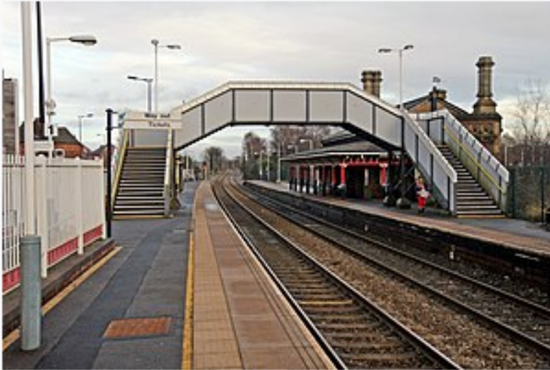
Earlestown station buildings viewed from platform 1
