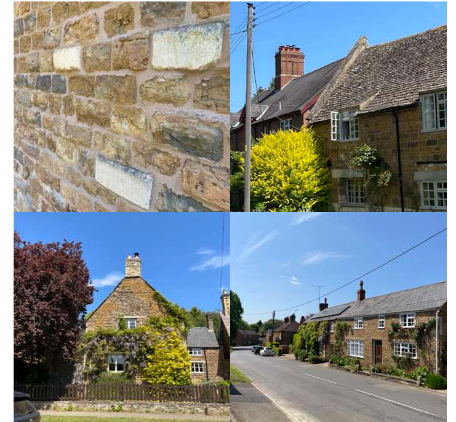
Iron stone, parapet gable ends, expressed gables and simple tiled roofs are common in the conservation area.
