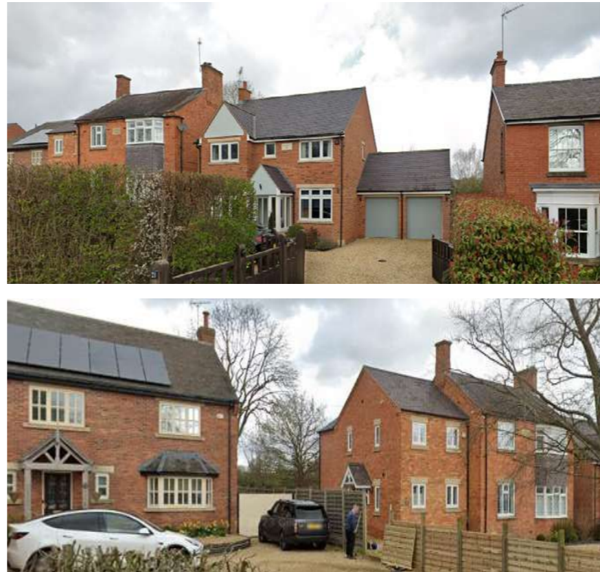
Examples of houses in immediate vicinity with minimal architectural value (©Google)
