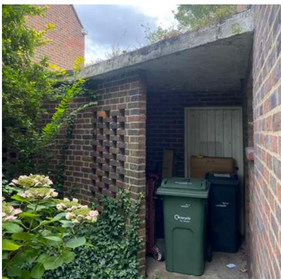
View towards the side outhouse – with concrete flat roof
