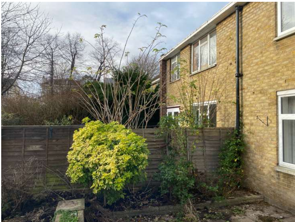
View of boundary with neighbour at No. 3
