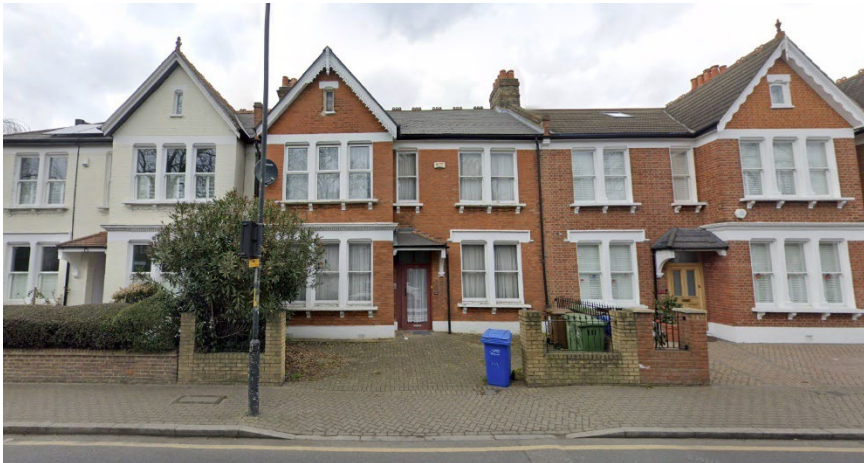
Front Elevation of 111 Half Moon Lane
