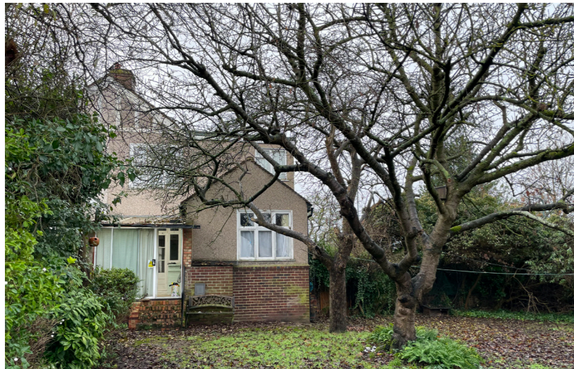
② Rear single storey extension
