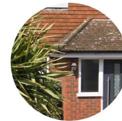
Red clay tiles with red brick
