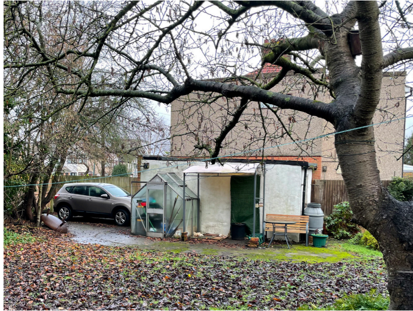
① Garage building
