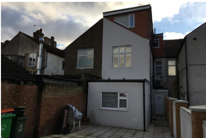
View from rear of No. 44 looking south
