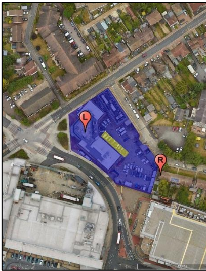
Figure 1 Aerial view of site (courtesy of Google Earth Pro). An indicative region showing the location of the proposed plant deck is highlighted in yellow
