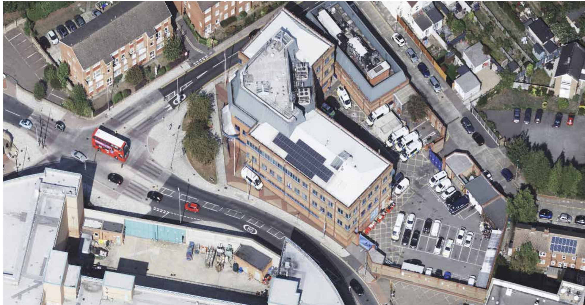
Existing aerial view of site showing roof and service yard/car park to rear of building.
