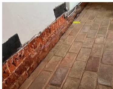
Removal of render exposed the delaminated bricks as marked by the red line below.
