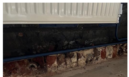
Removal of render exposed the delaminated bricks as marked by the red line below.
