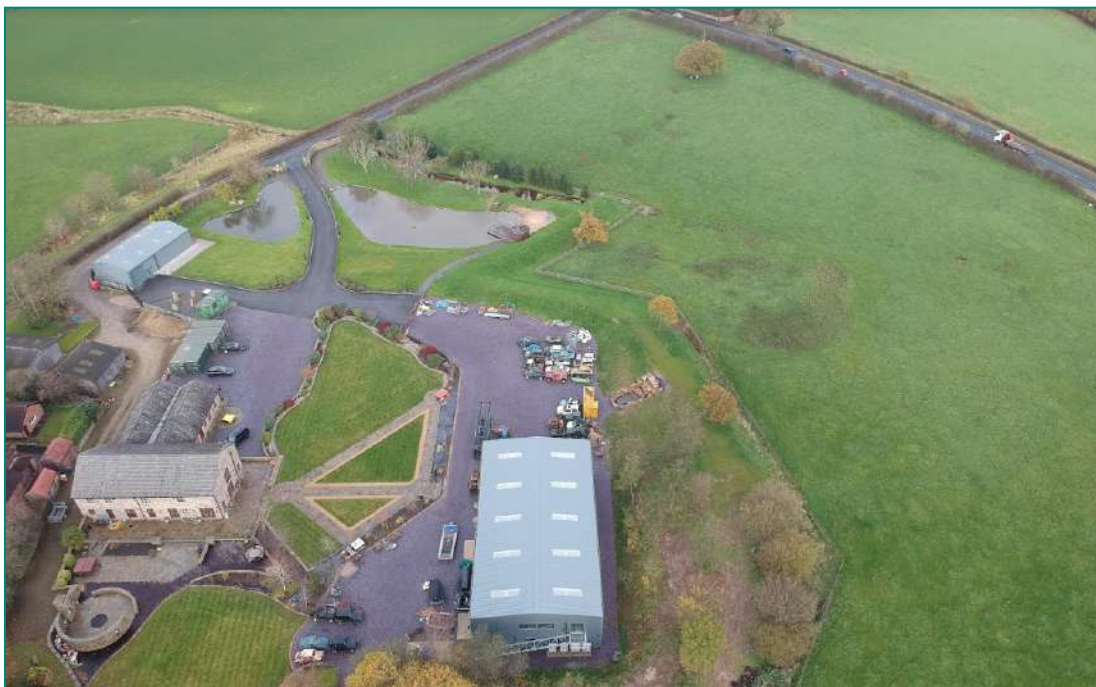
Figure 17 (Drone footage image 2023 with existing storage building)
