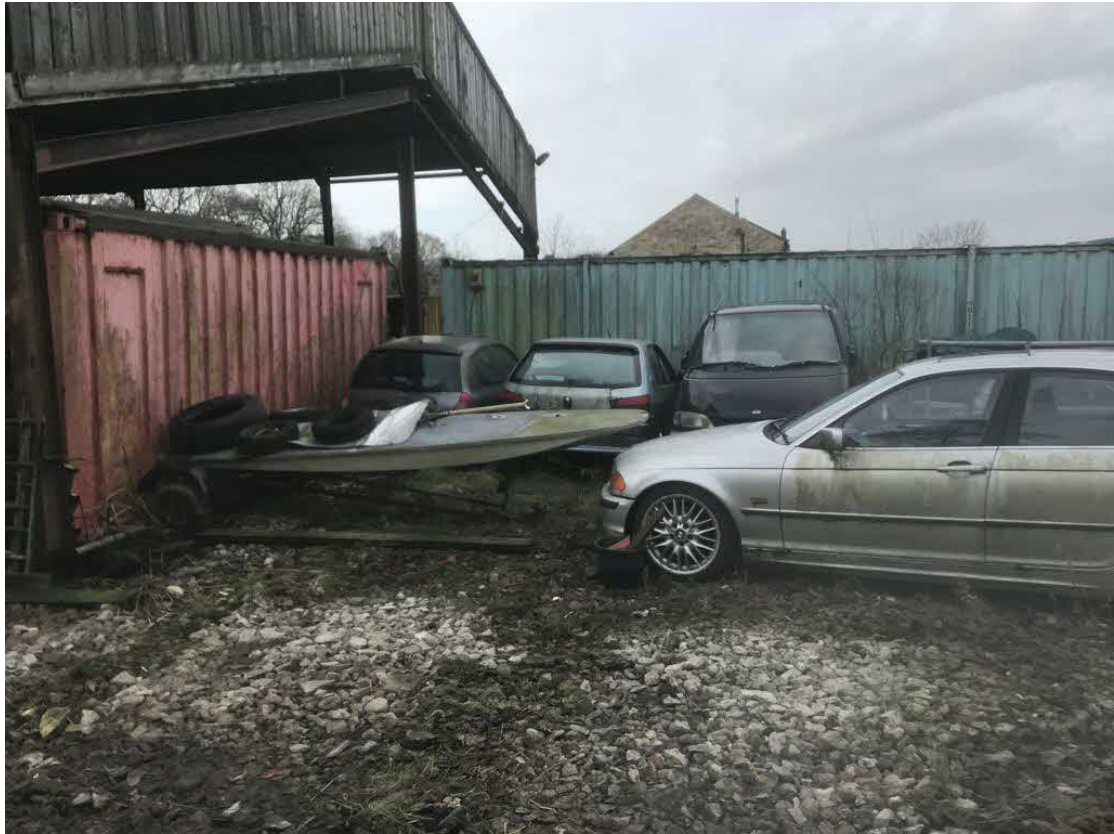
Note exposed slender beams and columns with extensive corrosion.
