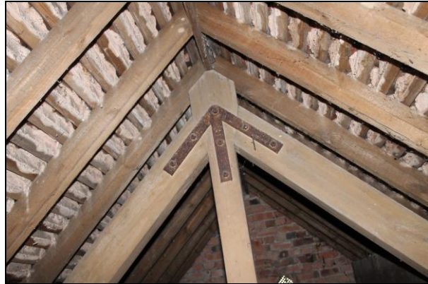
Plate 2:A: View of the underside of the northern roof
