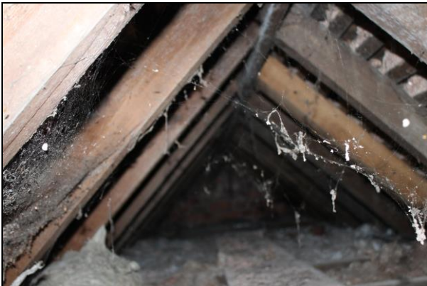
Plate 7:C: Interior view of the small loft space of the "Offices"
