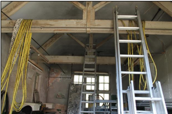
Plate 3:A: View of the interior of the central pitched roof section
