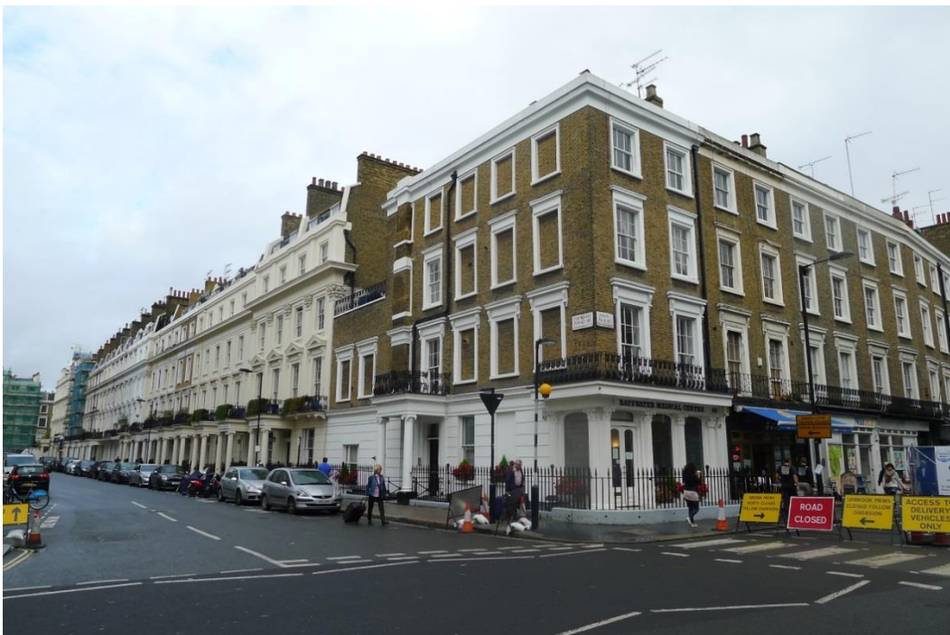
Figure 3.6: View looking North along Devonshire Terrace – 1850s terraces
