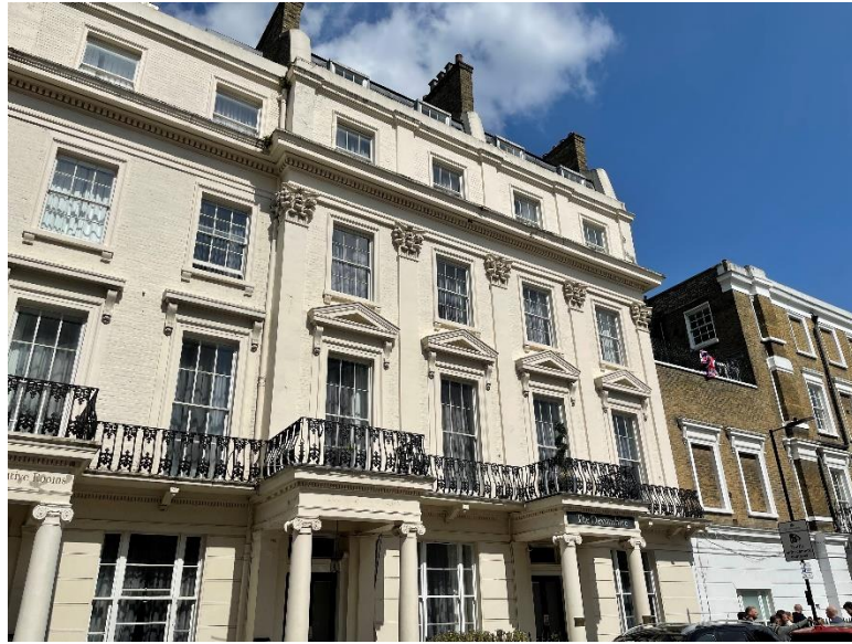
Figure 3.1: Nos.1-2 Devonshire Terrace
