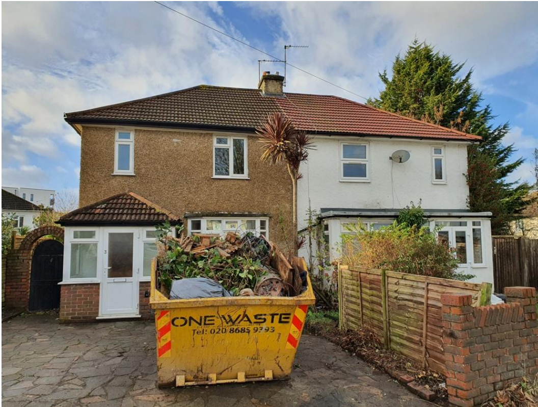
Front elevation view of subject property
