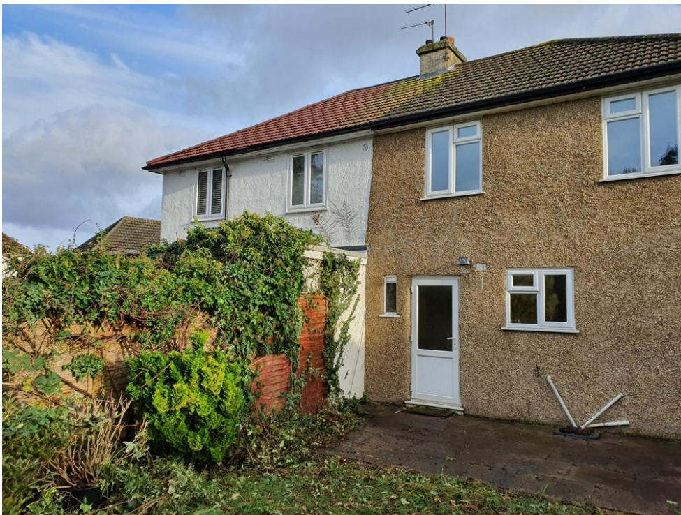
Rear elevation view of subject property
