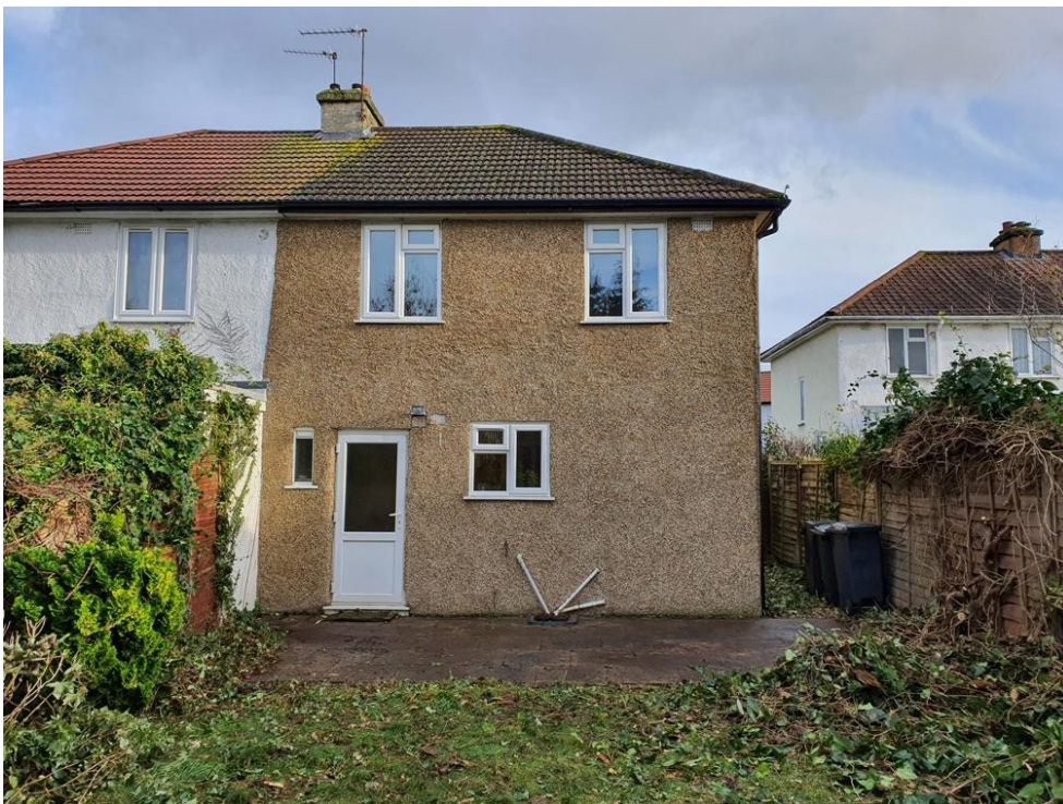
Rear elevation view of subject property
