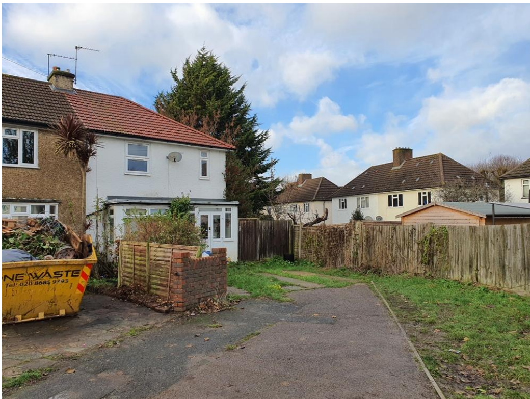
Front elevation view also showing the adjoining neighbouring property to the right side
