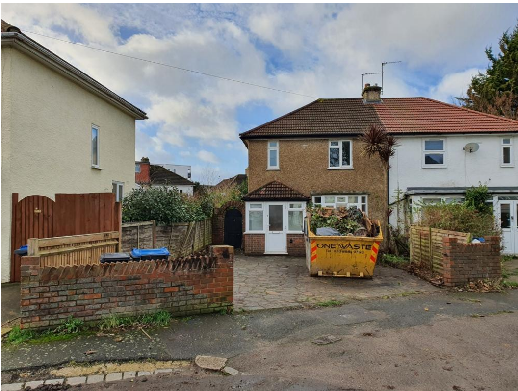
Front elevation view of subject property
