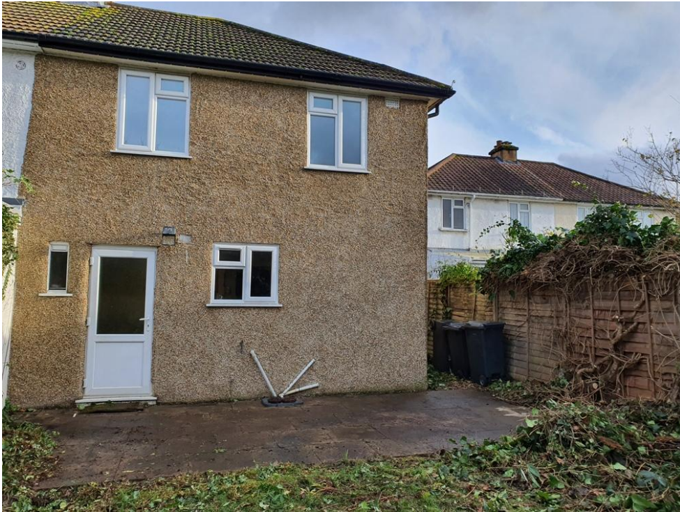
Rear elevation view of subject property
