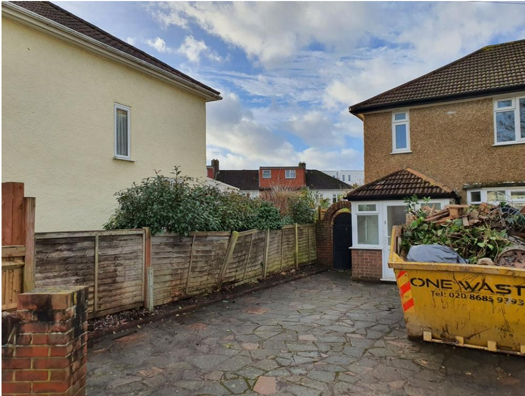
Front elevation view also showing the adjoining neighbouring property to the left side
