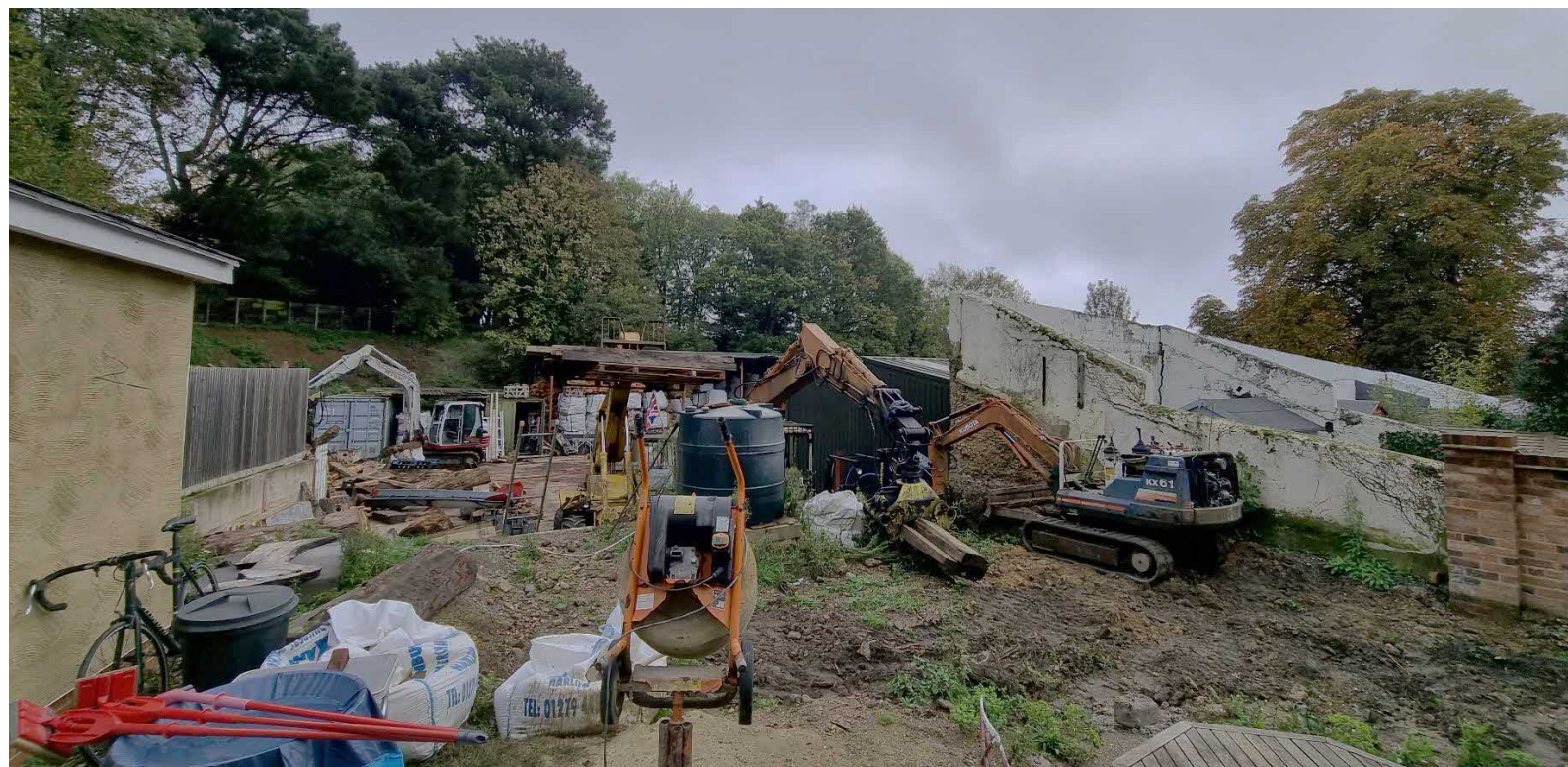
Figure 3: Rear of site and ground change
