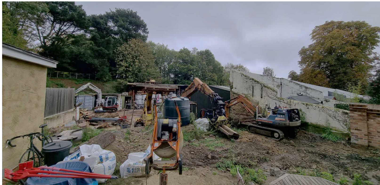
Figure 3: Rear of site and ground change
