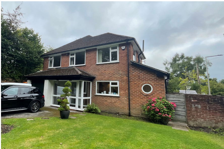
Figure 1: photo, 11 Robins Lane – main façade.
