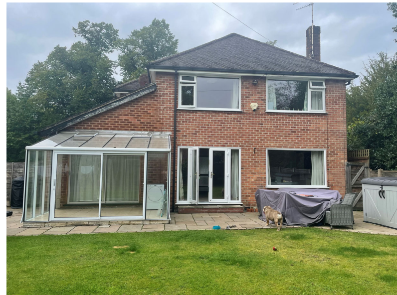
Figure 2: photo, 11 Robins Lane – rear façade.
