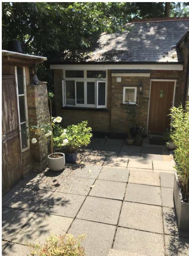
3 – Current access to the property is not visible from the approach and many visitors wander aimlessly around the site and enter in family areas.
