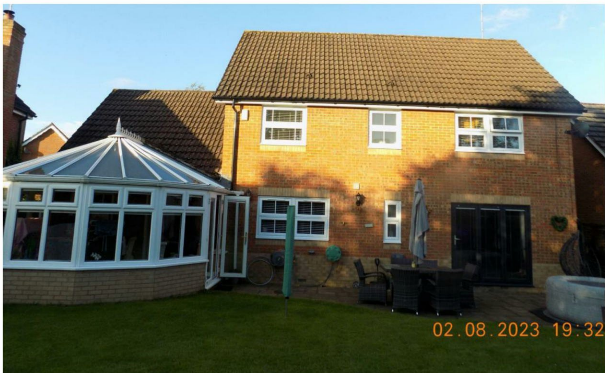
Image 2 – Rear West facing elevation of the property
