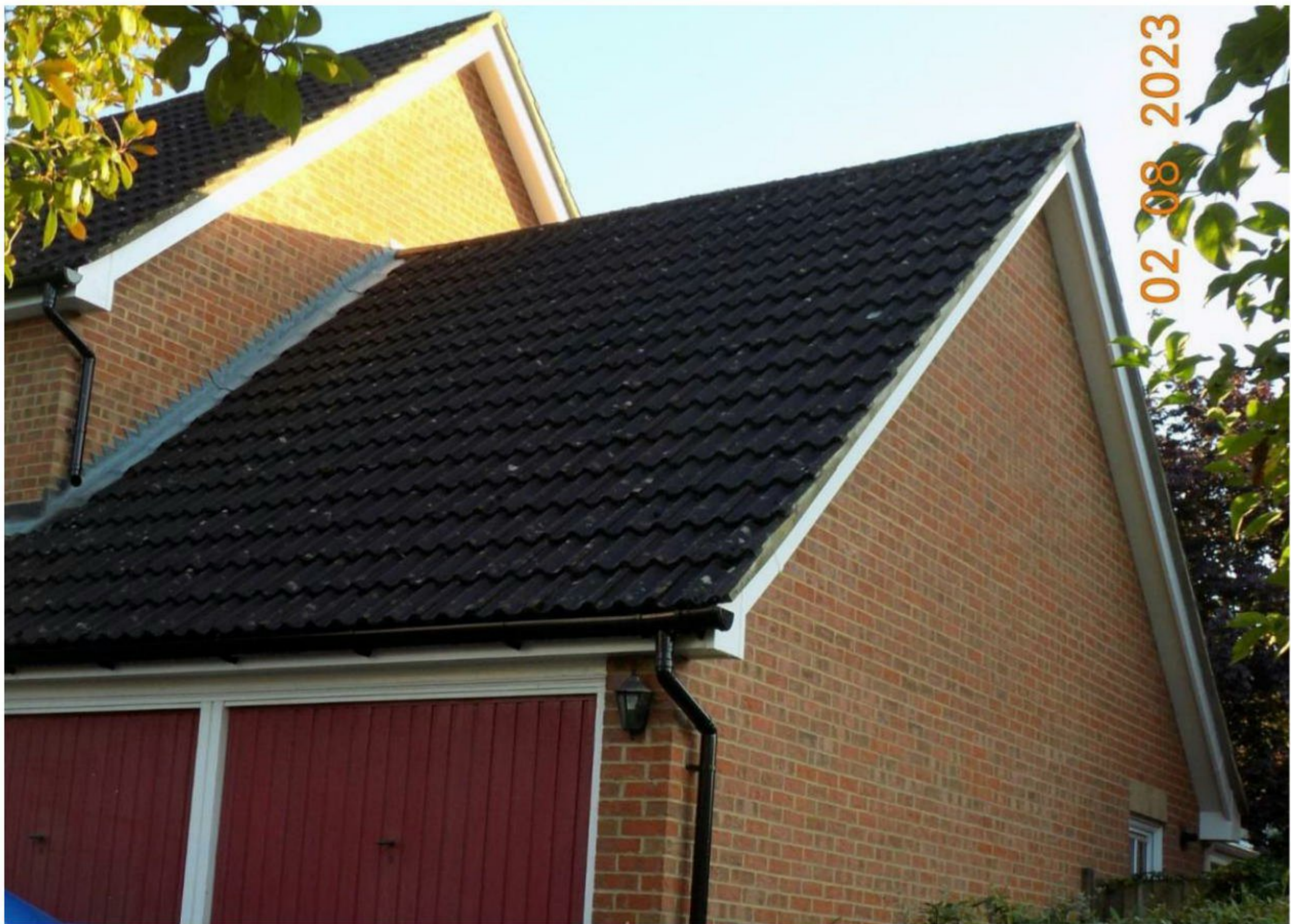
Image 3 – North facing gable elevation of the property
