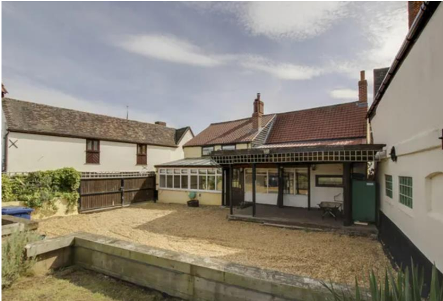
Plate 2: Photograph of the rear elevation of 49-51 Church Street
