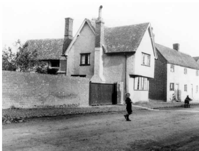
Figure 8: Historic photograph of Tudor House and 49-51 Church Street, 1920s
