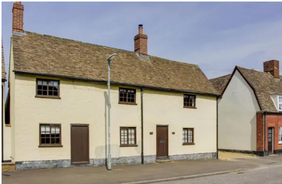
Plate 1: Photograph of the front elevation of 49-51 Church Street, Gamlingay
