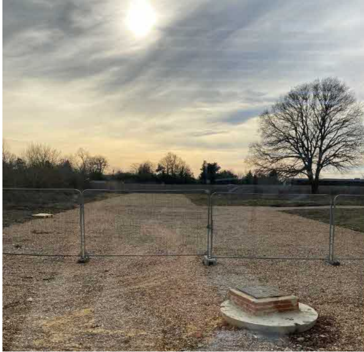
Fig2. Overflow car parking
