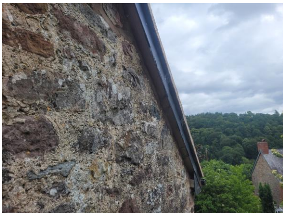
P5: Detail of the mortared rafter crevices
