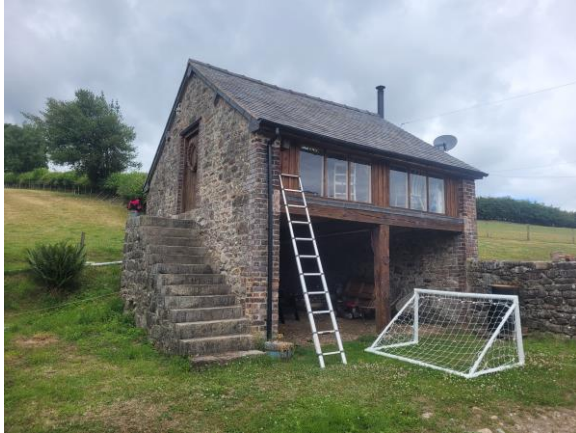
P1: S (gable) + E (side) elevations: looking NW
