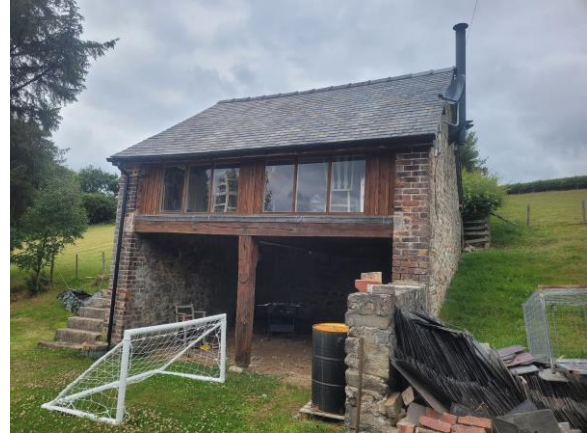
P2: E (side) + N (gable) elevations: looking SW
