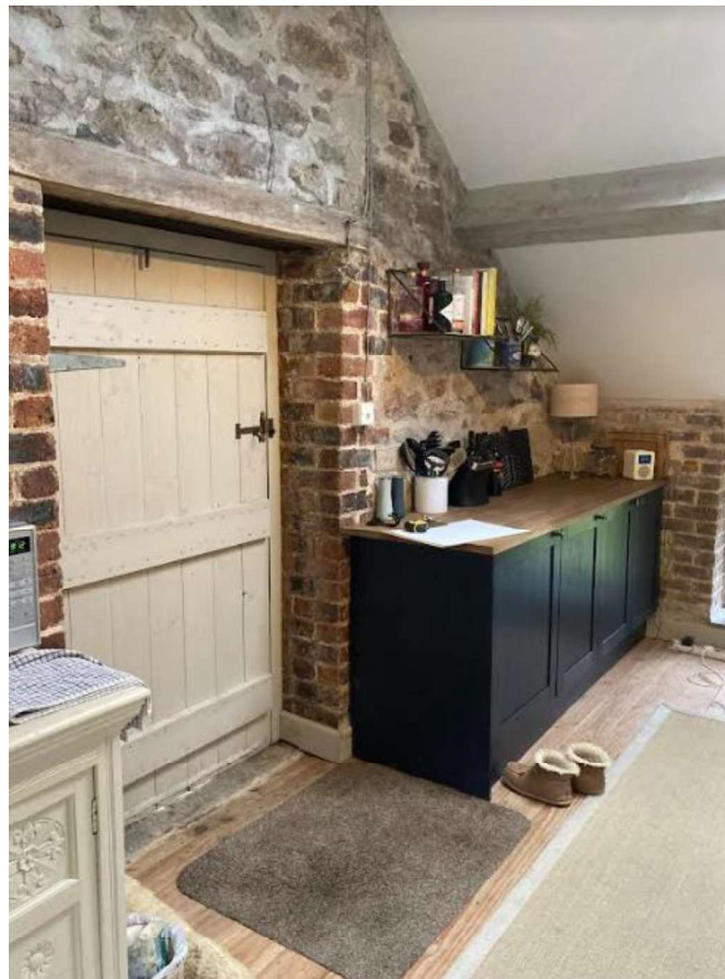
Pl.4: Part of the interior of the restored loft or granary floor.
