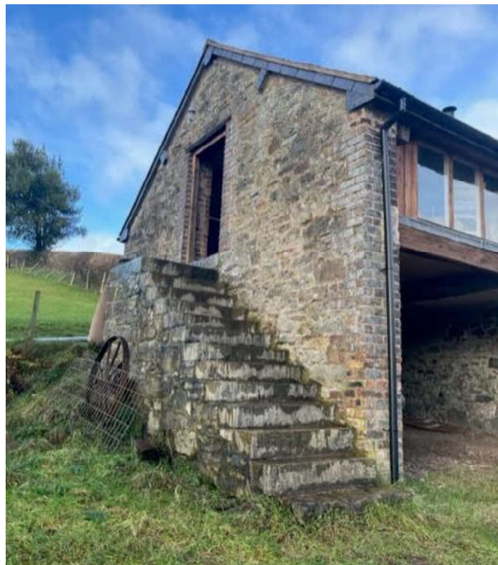
Pl.3: The south gable of the Cart Shed.
