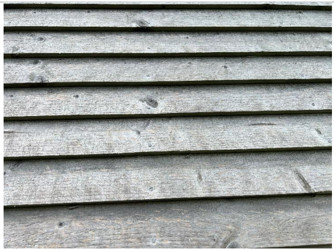
Part cladding at north elevation
