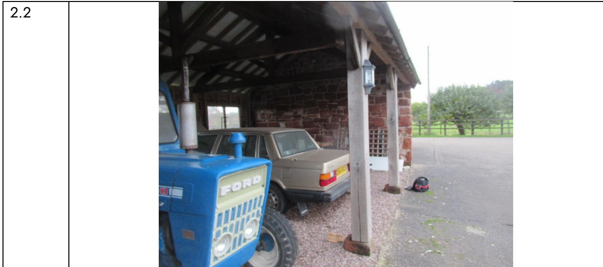
Supporting beams for frame
