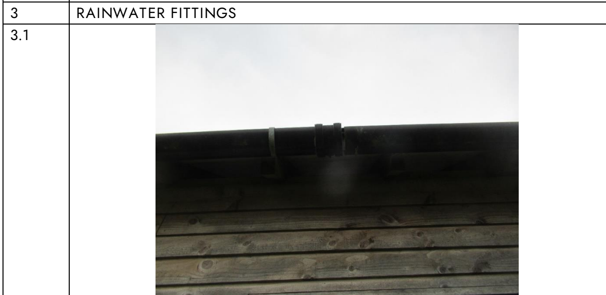
Disconnected gutter joint
