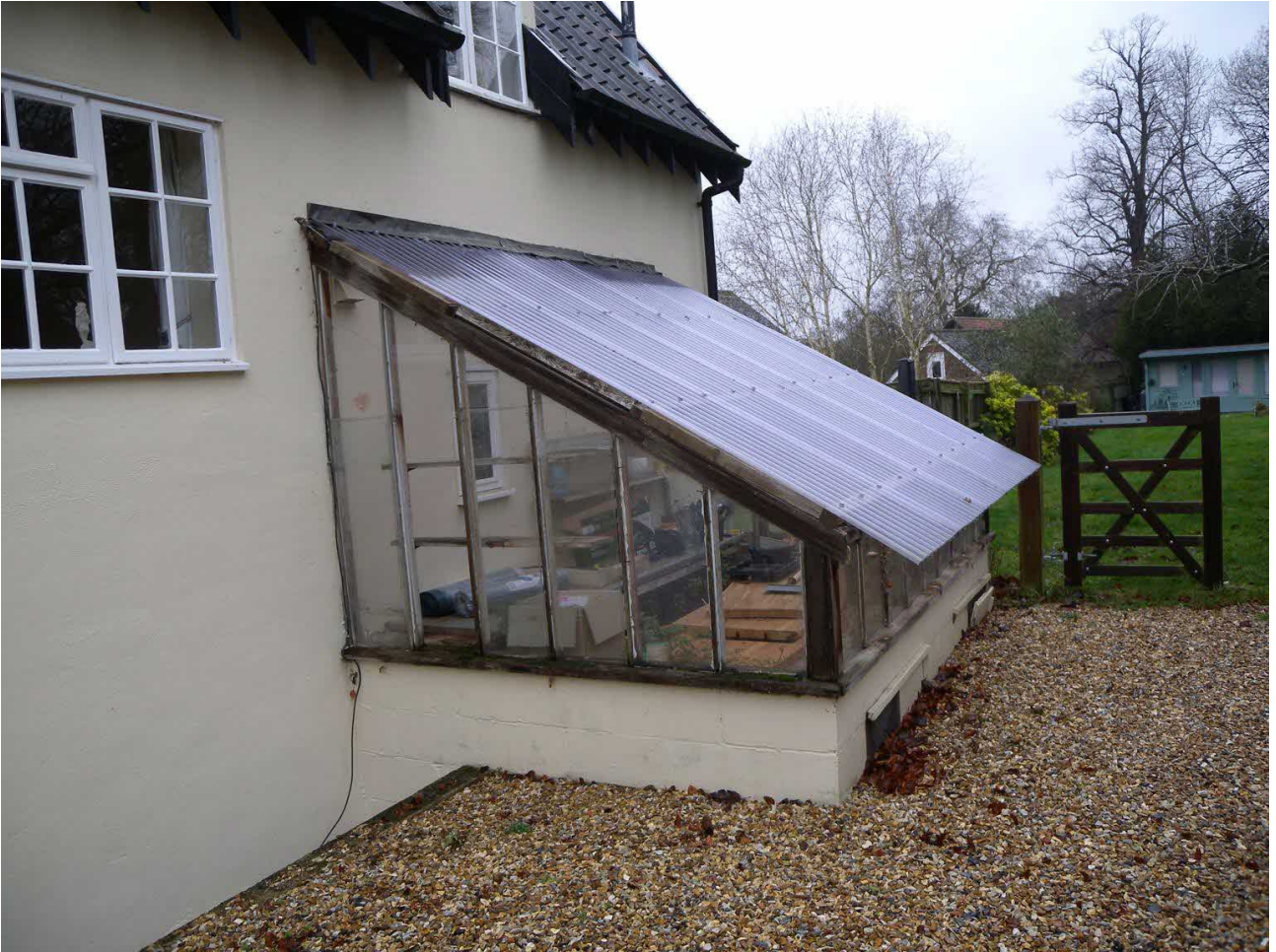
Abbots Lodge - Building C Glass Lean-to
