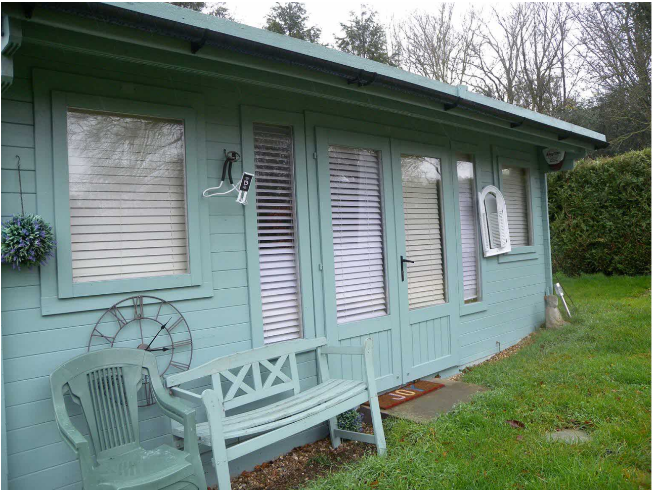
Abbots Lodge - Building A
