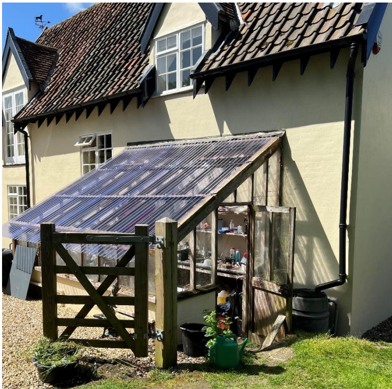
Figure 4 : showing existing lean-to glass house.
