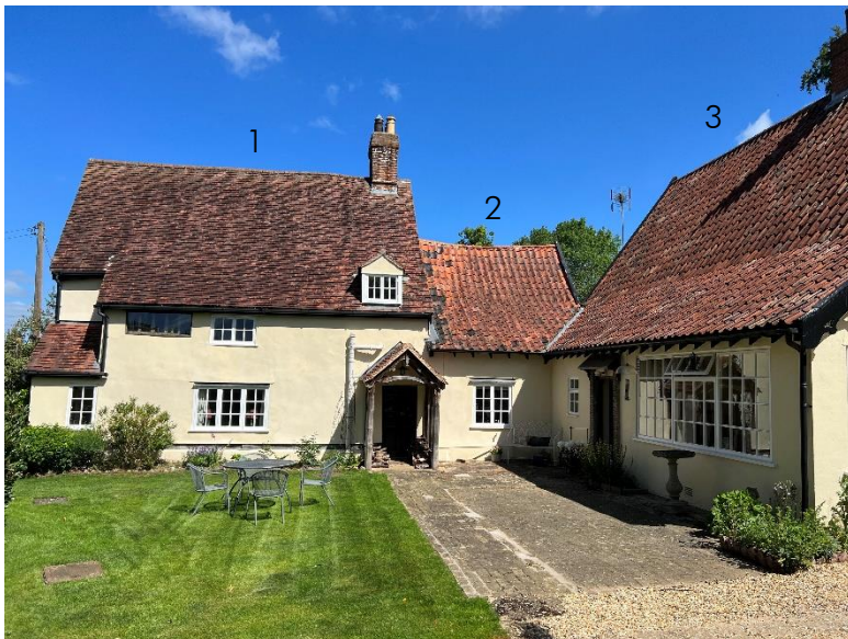
Figure 6 : showing South façade of the historic building described in the listing with, from left to right :
