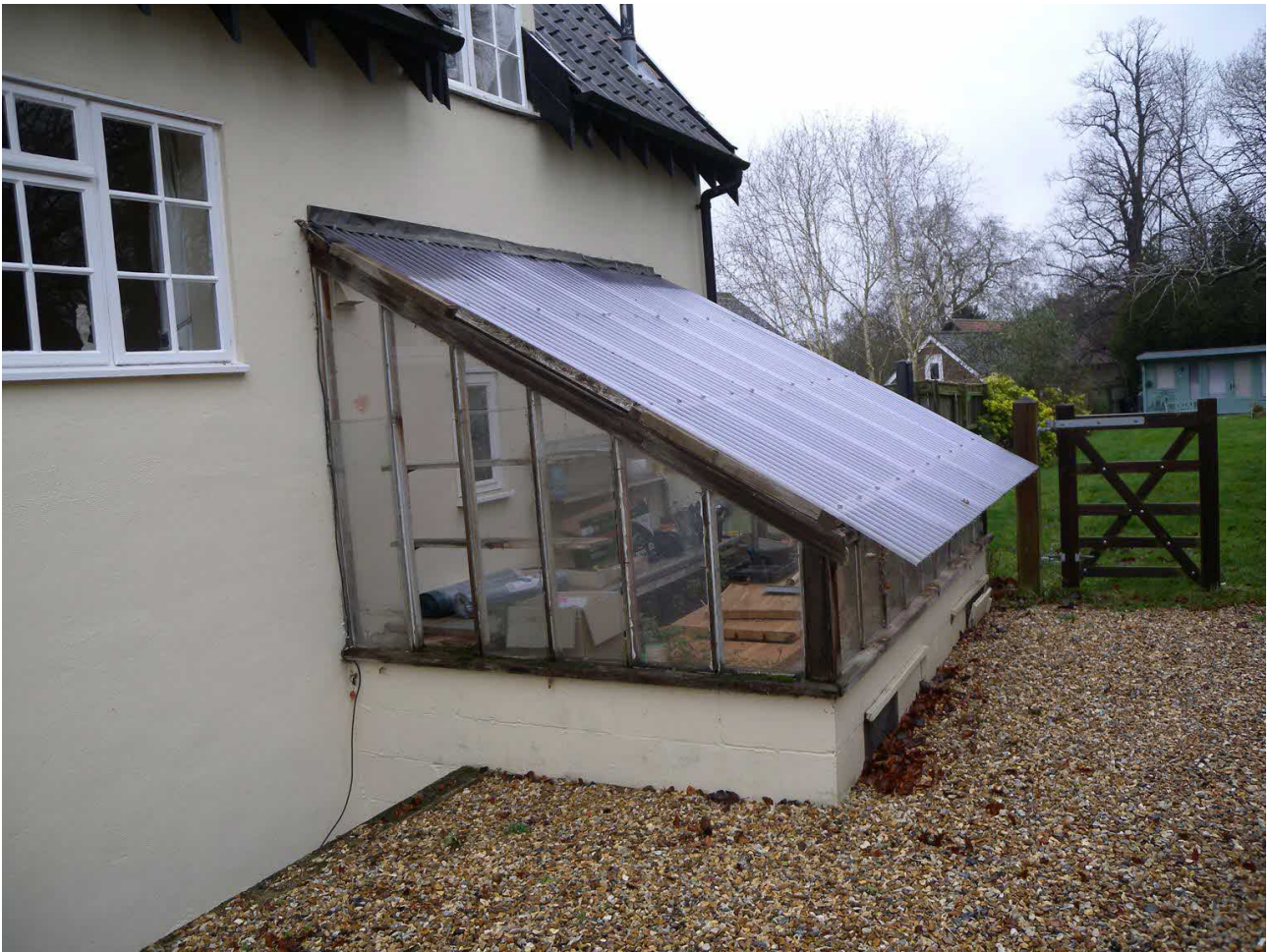
Abbots Lodge - Building C Glass Lean-to
