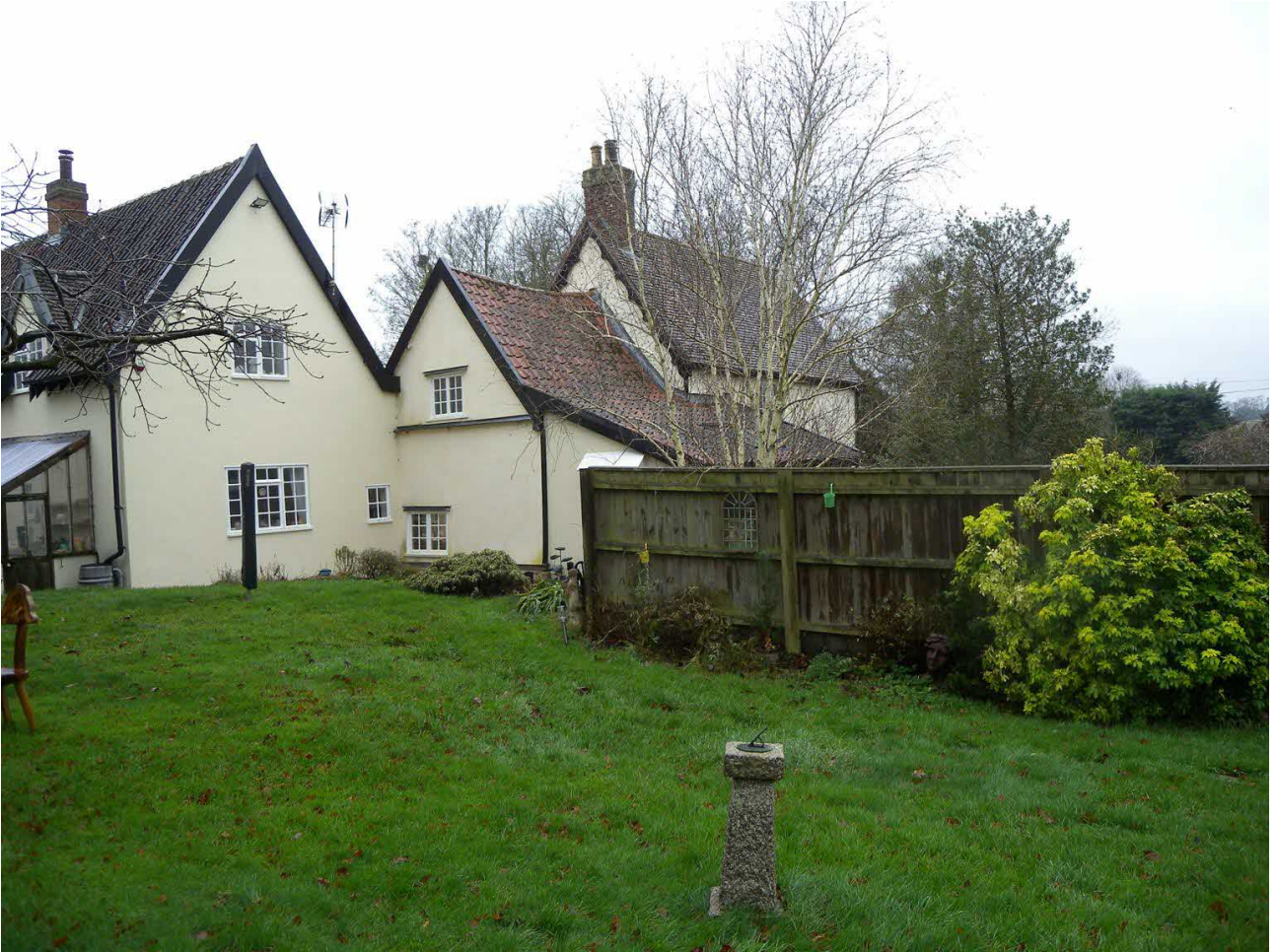
Abbots Lodge - NE face of buildings B and C
