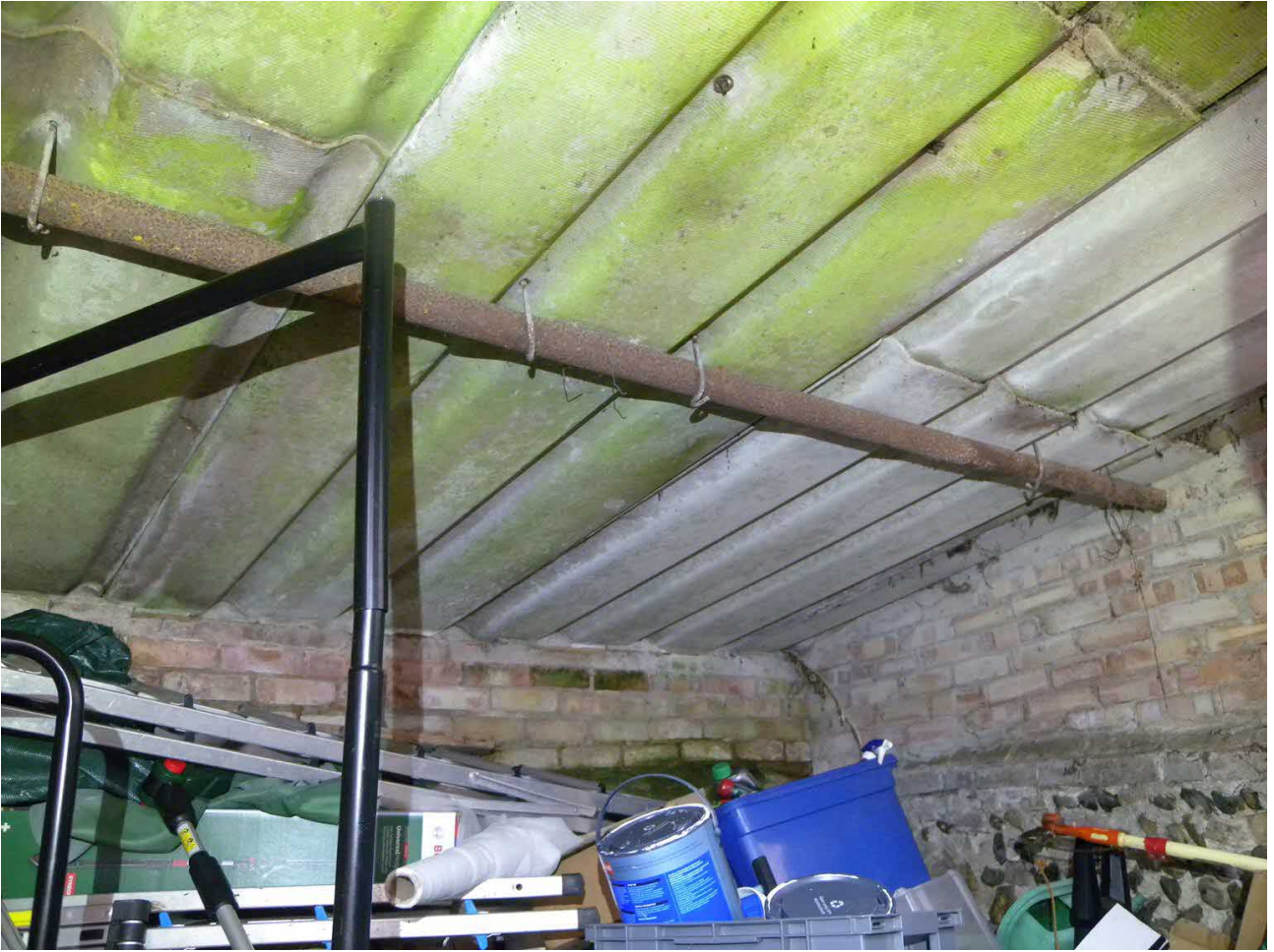
Abbots Lodge - Building D interior
