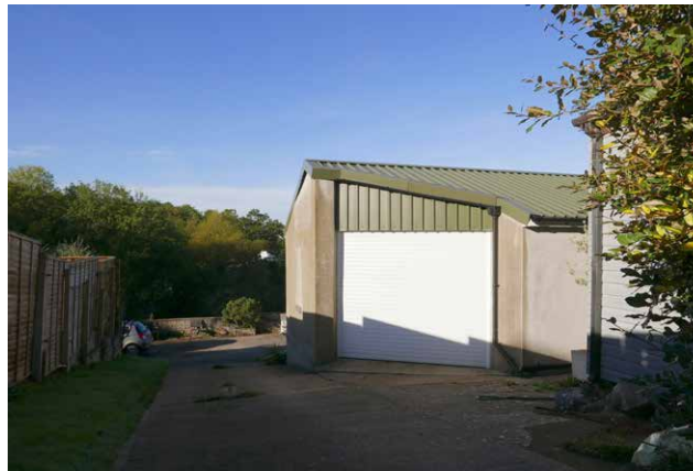
View of entrance to large outbuilding and sets out the reasons for making them.
