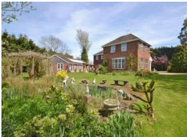
Photograph of West Elevation
