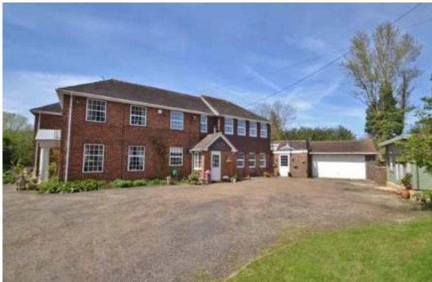
Photograph of East Elevation
