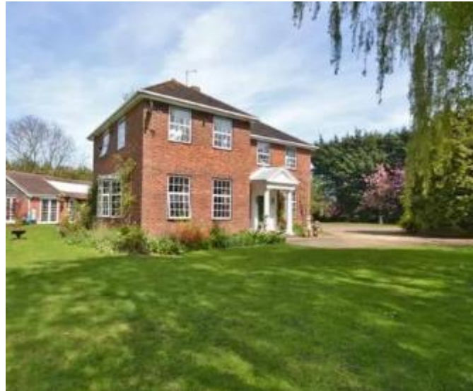
Photograph of Southern Elevation
