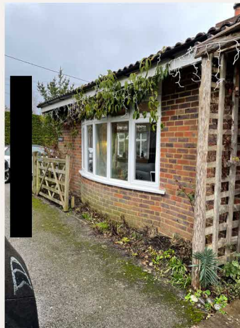
Existing front entrance
