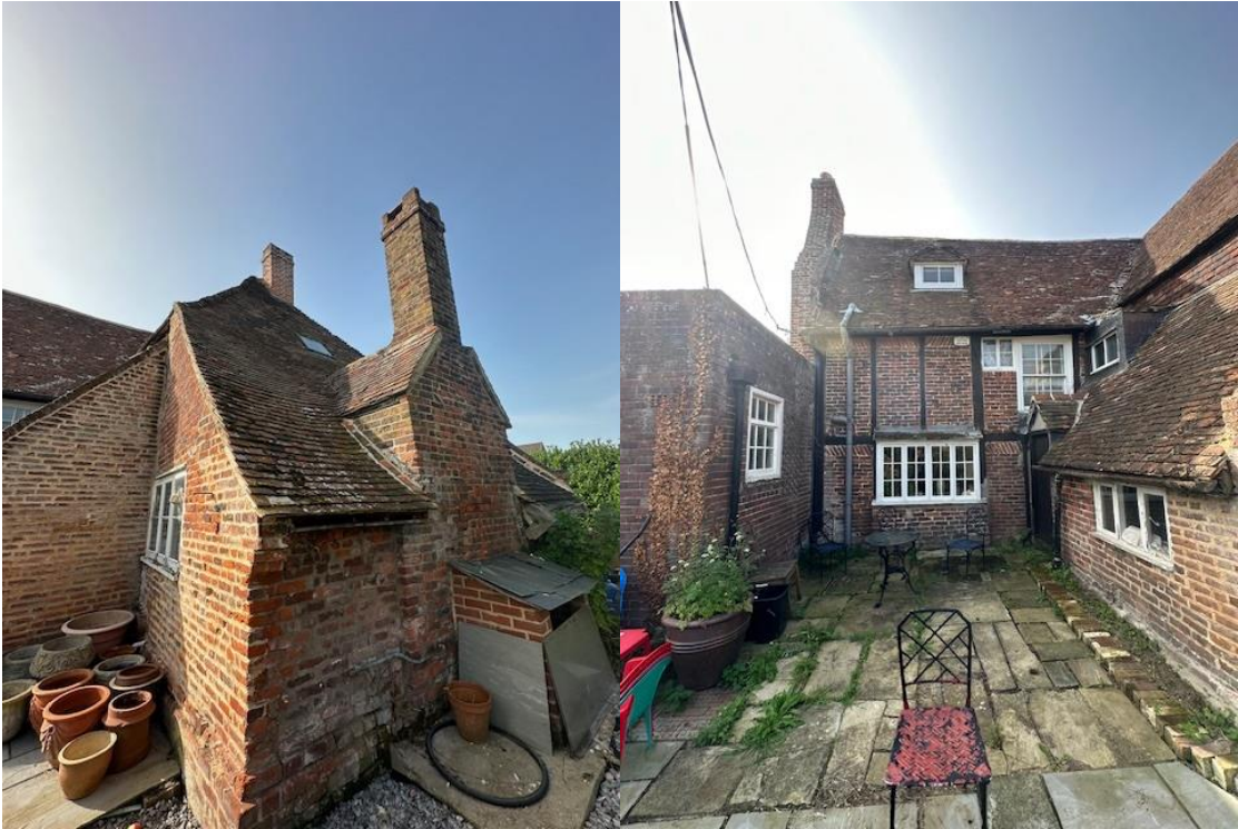
Existing rooflight window
