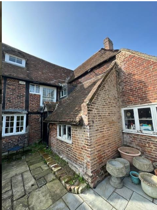
External view of existing window
