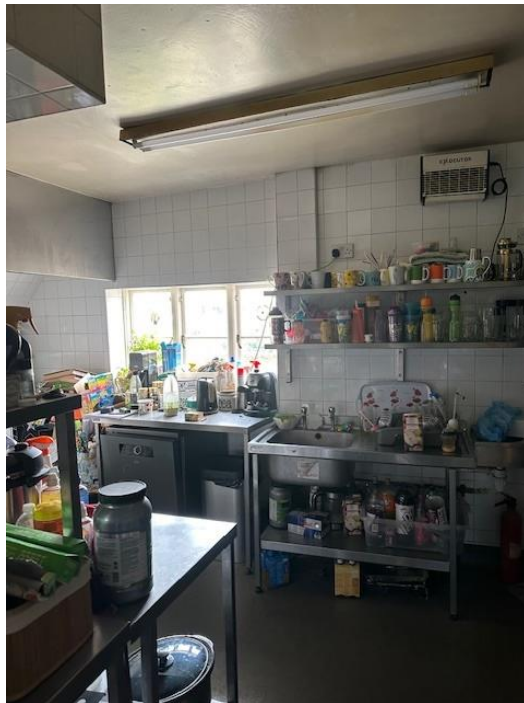
Internal view of existing window
