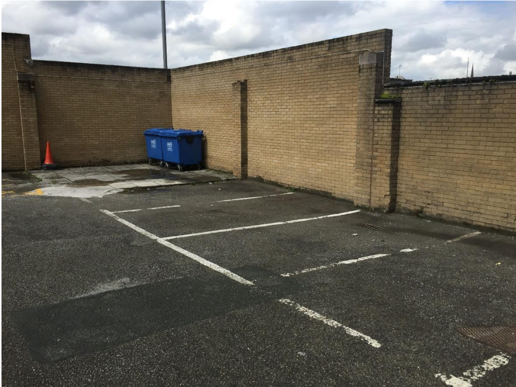
Fig 2. View into northwest corner (note: falls)
