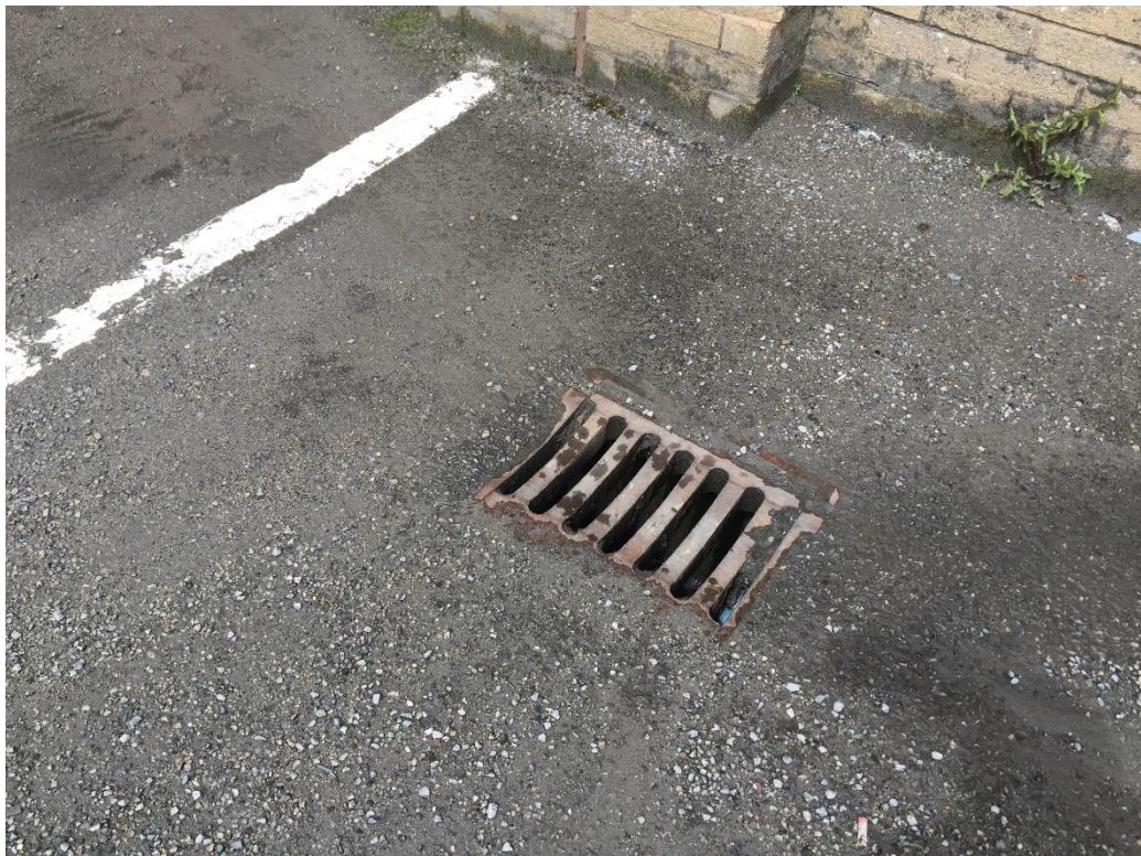
Fig 3. Storm water gully in parking space no.3
