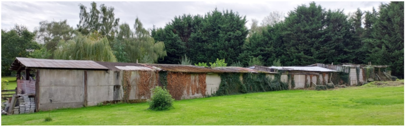
Photo of Existing Outbuilding
